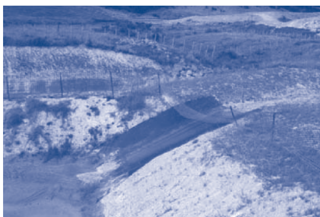
Example of a lined channel used to transport water down slopes and batters without eroding them.
