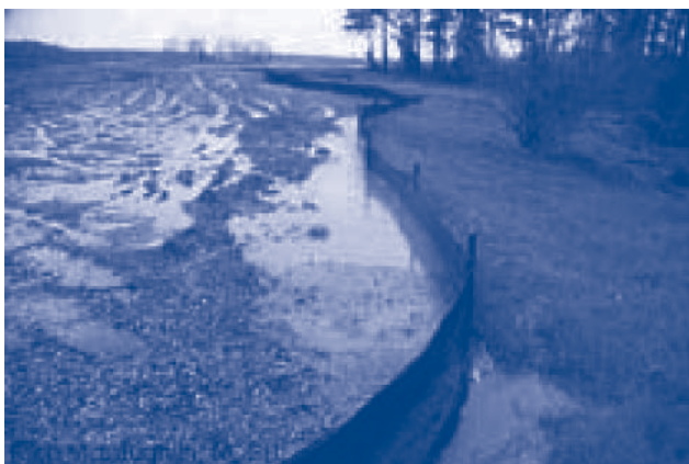
Example of sediment fencing installed along a site perimeter.
