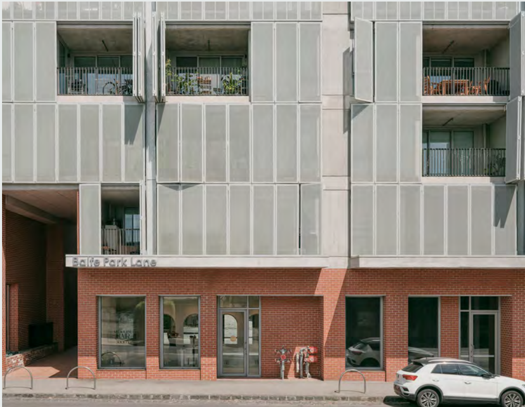
21.05 Perforated screens offer flexibility, balancing passive surveillance and street activation with privacy.
