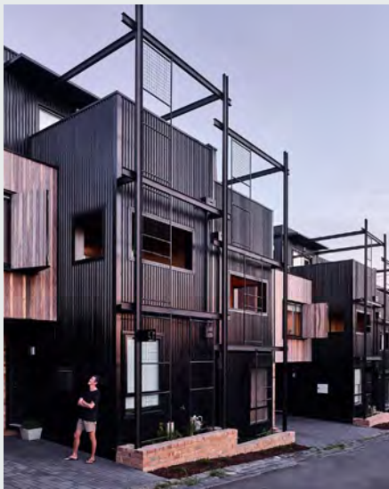
3.02 (left), 3.03 (right) An external mesh frame supports flowering vines.
