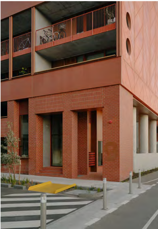
27.07 (top left) 27.08 (top right) 27.09 (left) 27.10 (right) Integrated landscape architecture and material expression reinforce the identities of each building.
