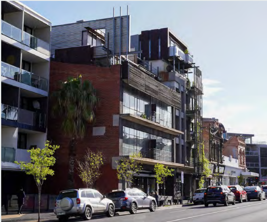
19.01 The facade incorporates a timber batten screen that supports climbing vines.
