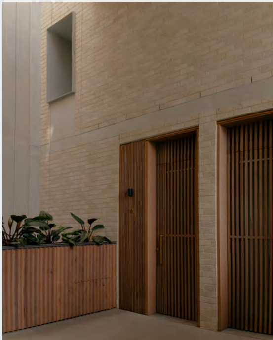
12.01 Balconies span the building facade incorporating hit and miss brickwork.
