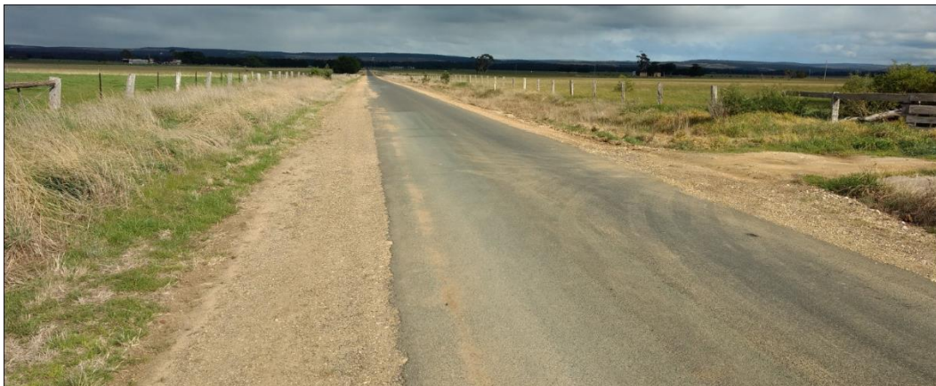
Figure 2-10 – East of the Site: Hopkins Road looking south
