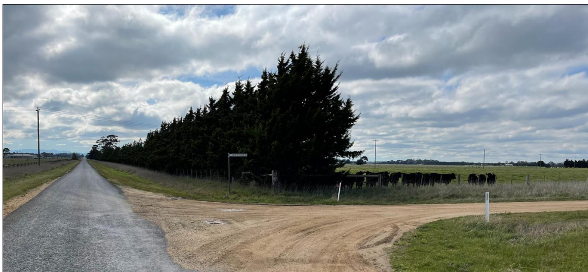
Figure 2-7 - 66KV Powerline intersecting Settlement Road (corner of Lower Settlement Road)
