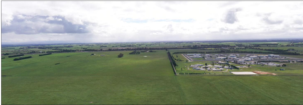
Figure 2-9 - View from north-east of the site. Fulham Correction Centre located to the right of the image
