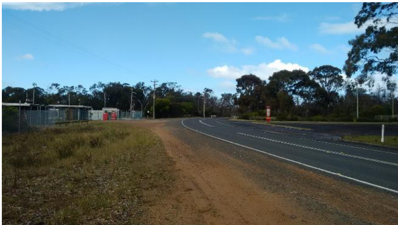
Figure 5: Support buildings associated with the Crib Point Jetty (source: Jacobs)
