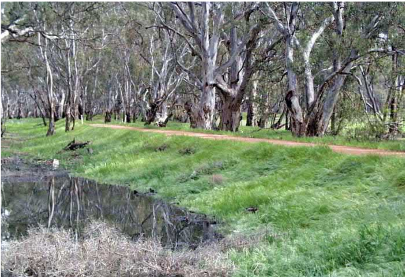
Figure 2.7: Takasuka Levee Bank (HO186 / NT B6238), located within the Vinifera State Forest, Forest / Takasuka Road reserve, and part of the immediately adjacent farmland (Allom Lovell and Associates 2001c, p. 501)
