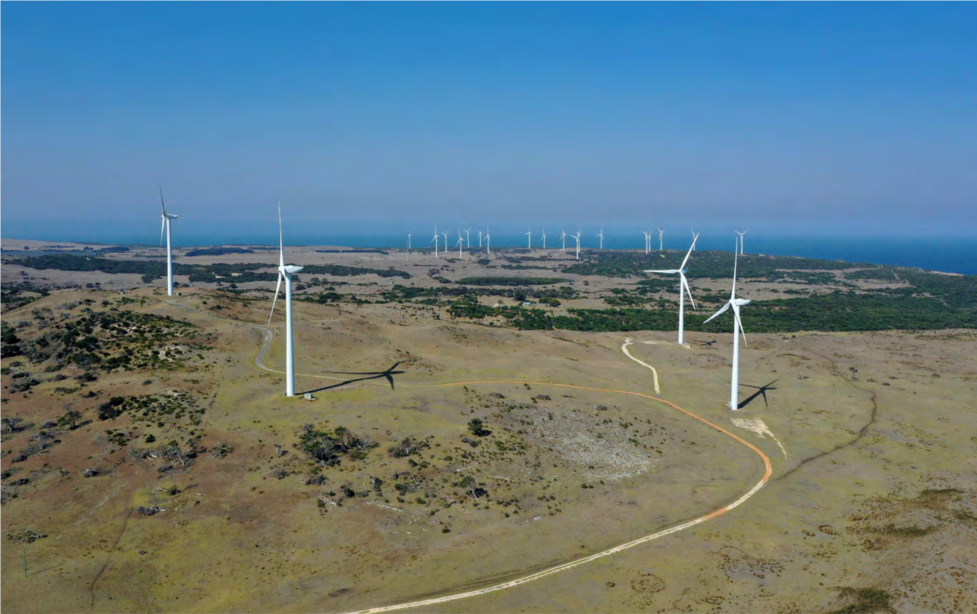
Aerial Photo from Amos Road, view south toward Cape Bridgewater
