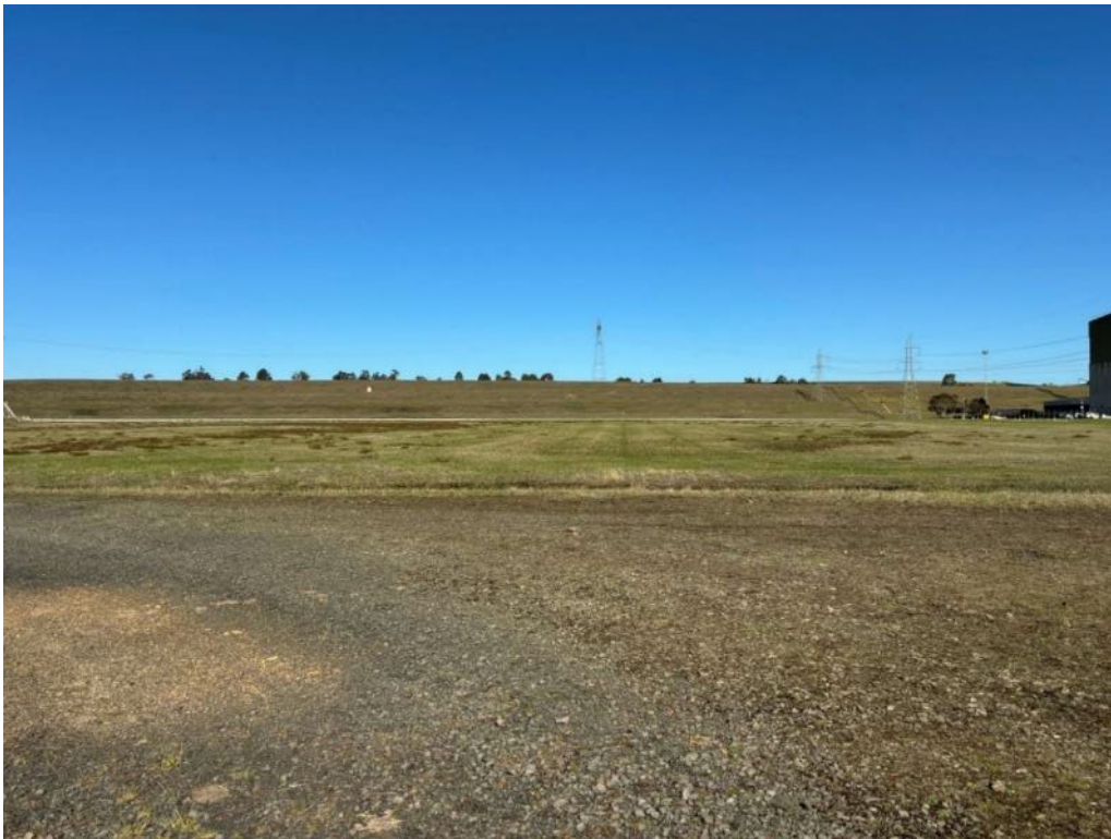
Plate 3 View of Activity 2 site facing south
