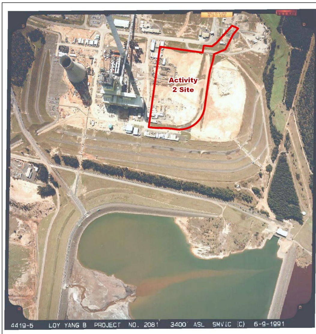
Figure 8 Aerial image from 1991 showing major earthworks in the northern section of the Activity 2 site (Landata)
