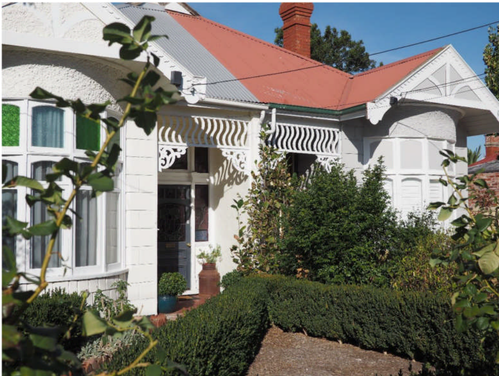
2 and 4 Ngarveno Street, Moonee Ponds, principal elevation (source: Context 2018)
