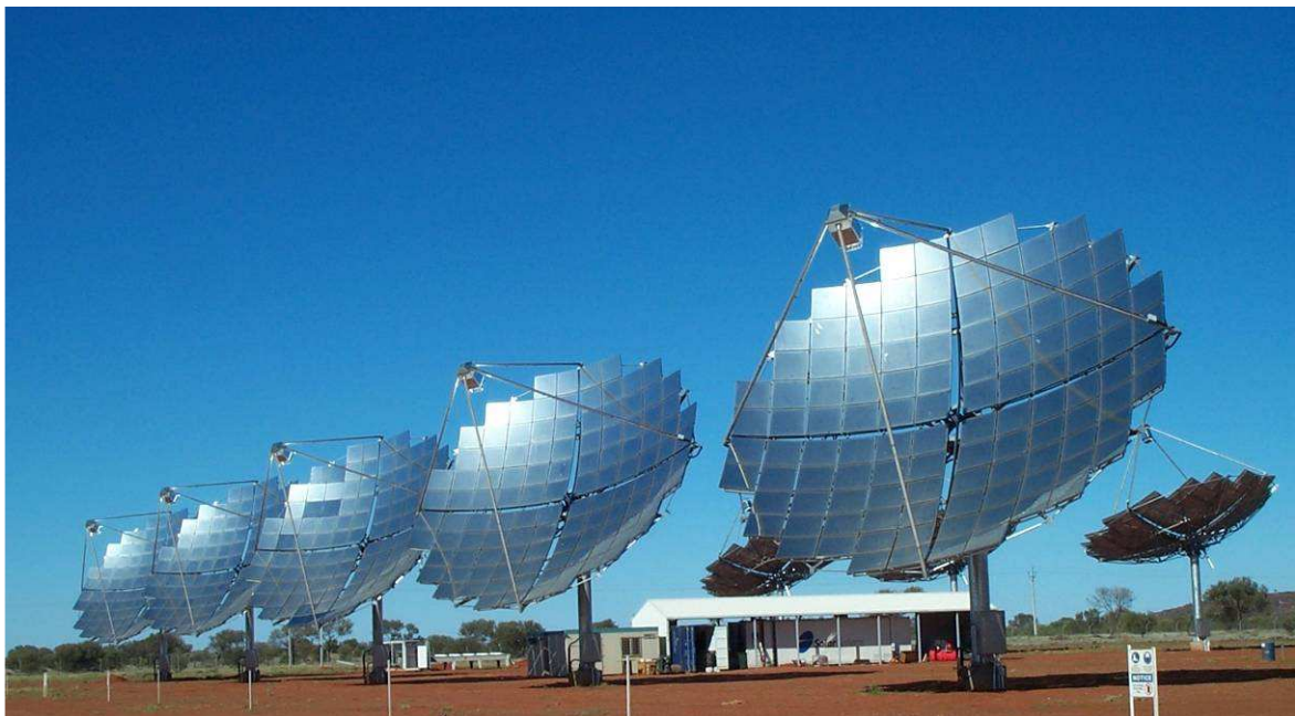
Solar Systems power station in remote central Australia
