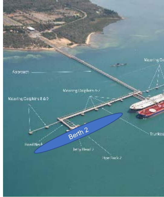
Figure 3: View of Crib Point jetty from the south-east
