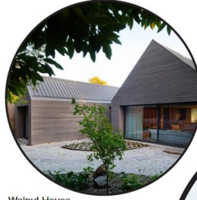
Walnut House Central Springs Rd, DAYLESFORD Adam Kane Architects
