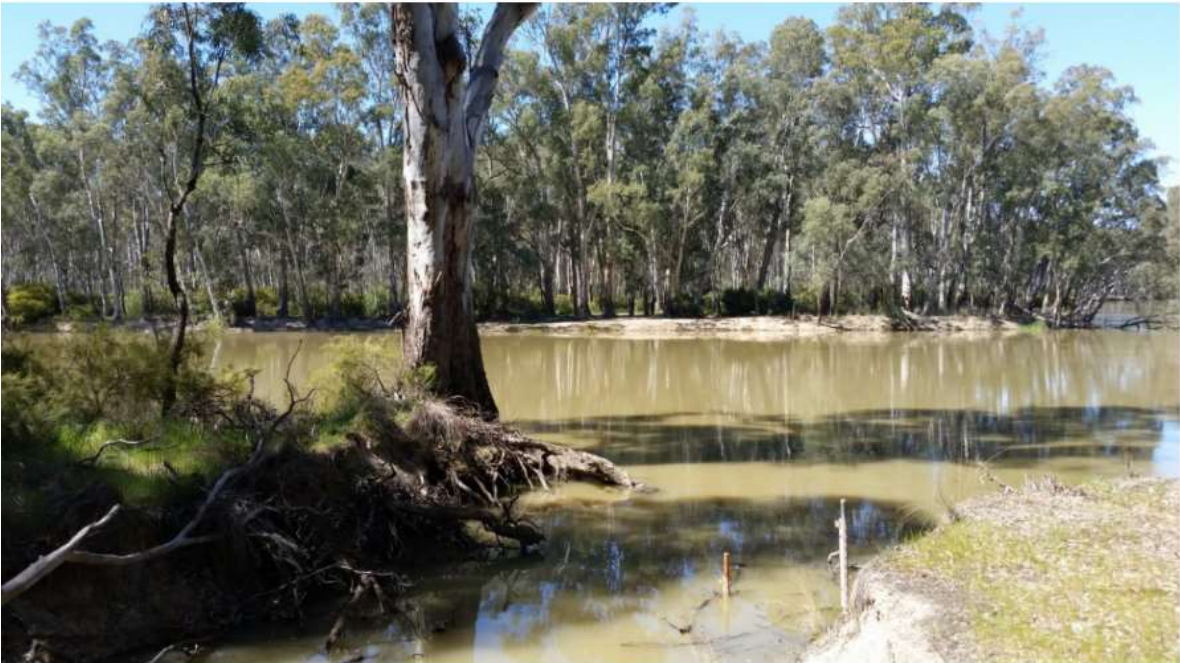
Figure 5 - Guttrum Main Outfall Drop Structure Site
