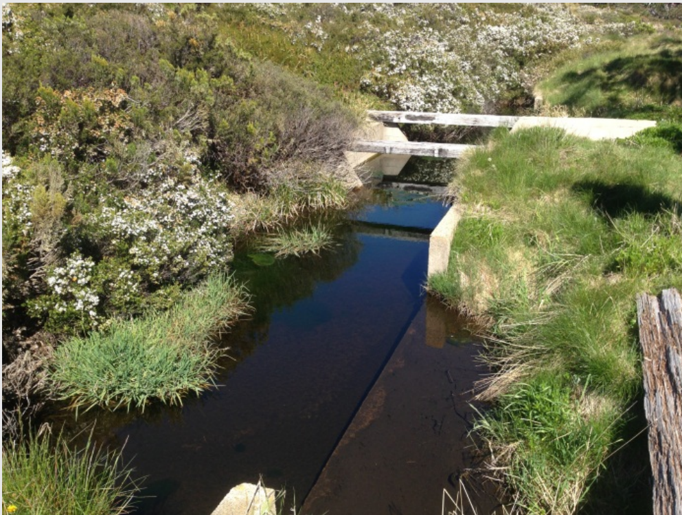
Photo taken of the aqueduct weir located west of BH7 along aqueduct
