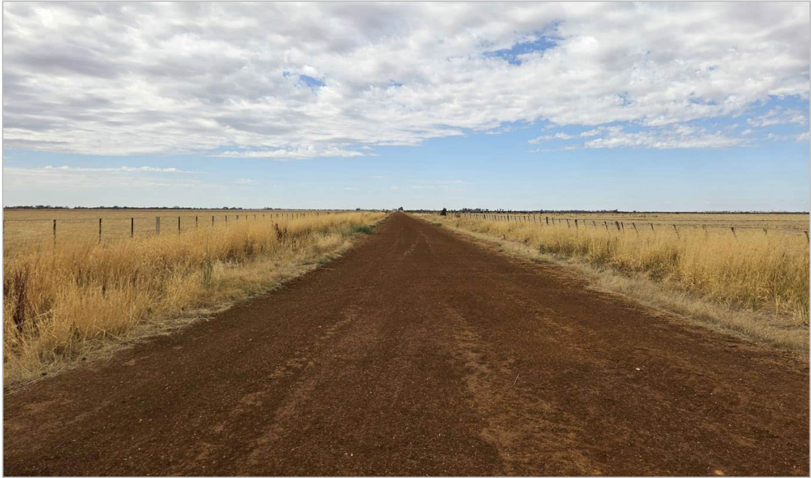
Figure 33: Typical Dry Weather (Dirt) Road – Grogan Road
