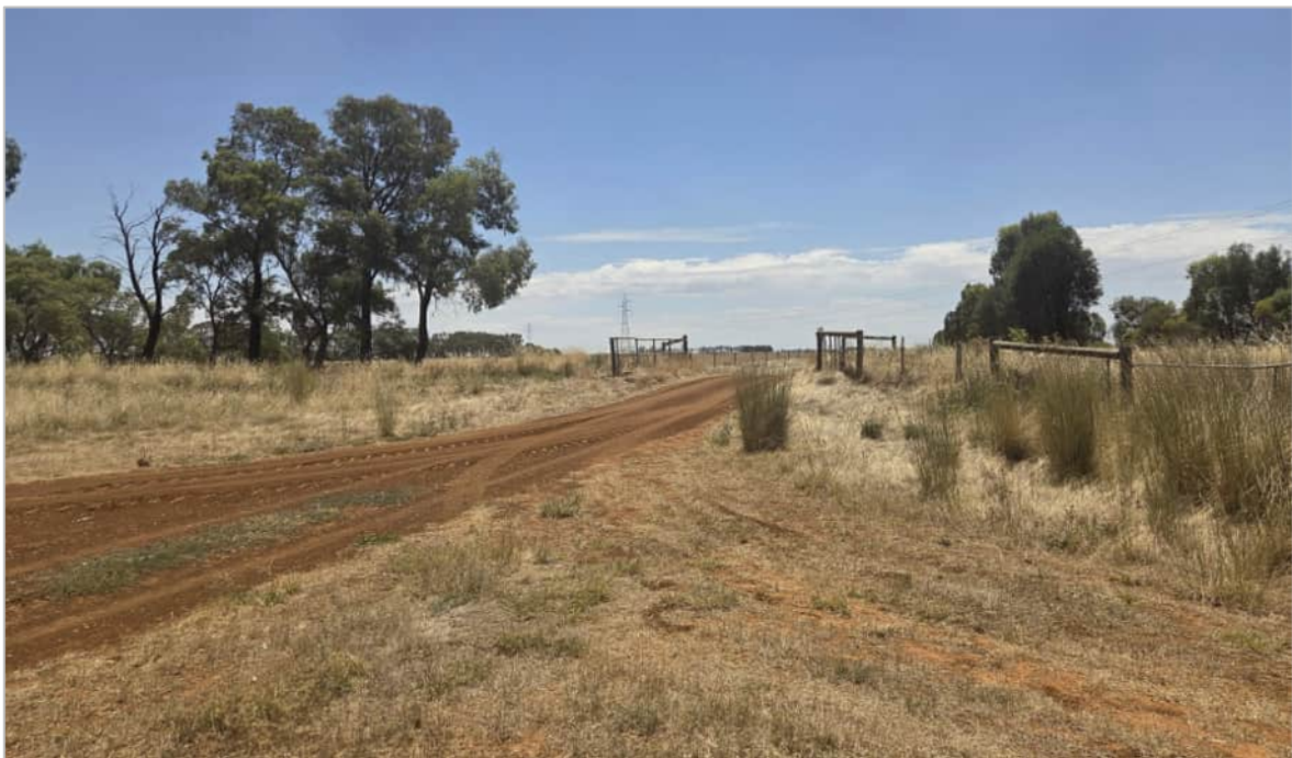
Figure 39: Restricted Sight Distance on Godwards Road
