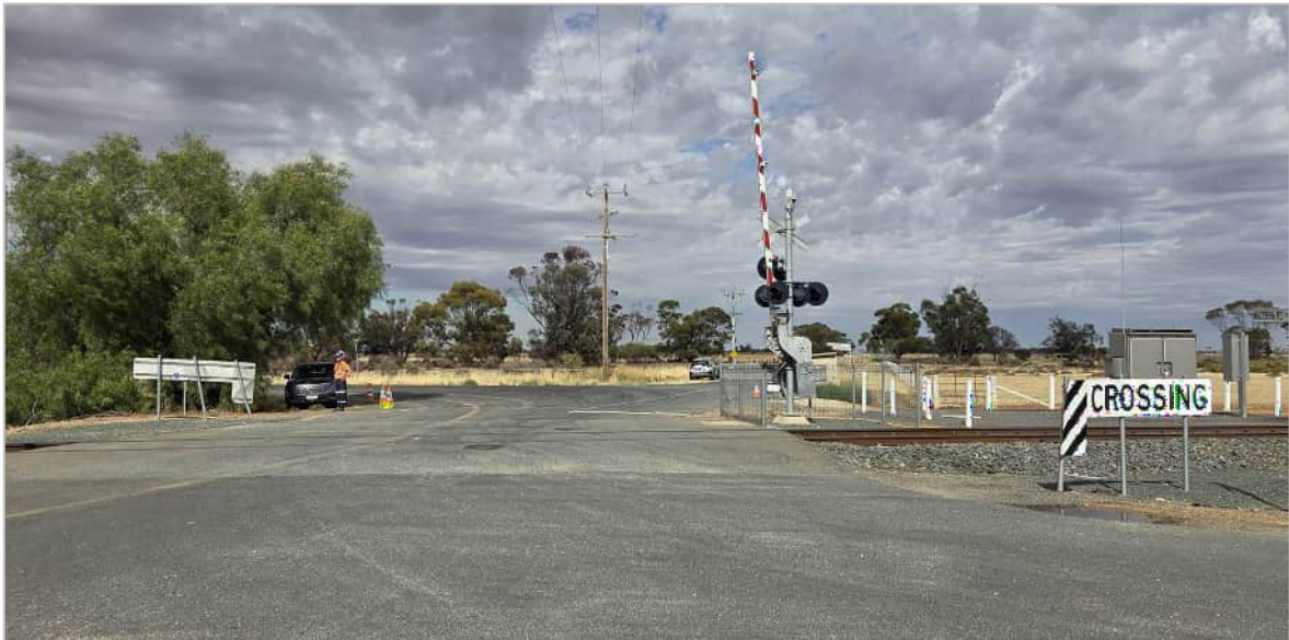
Figure 38: Restricted Sight Distance on Macorna Road
