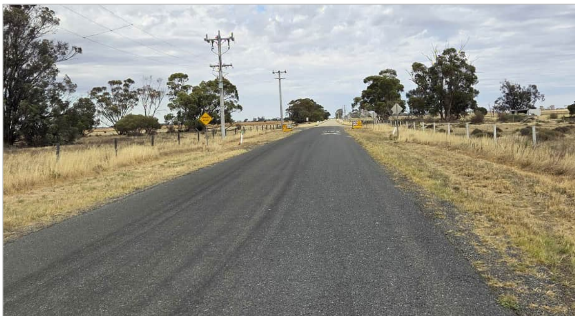
Figure 35: Typical Sealed Road – Kerang-Macorna Road
