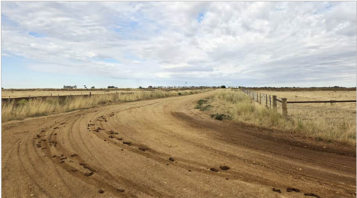
Figure 36: Restricted Sight Distance on Wishart Road
