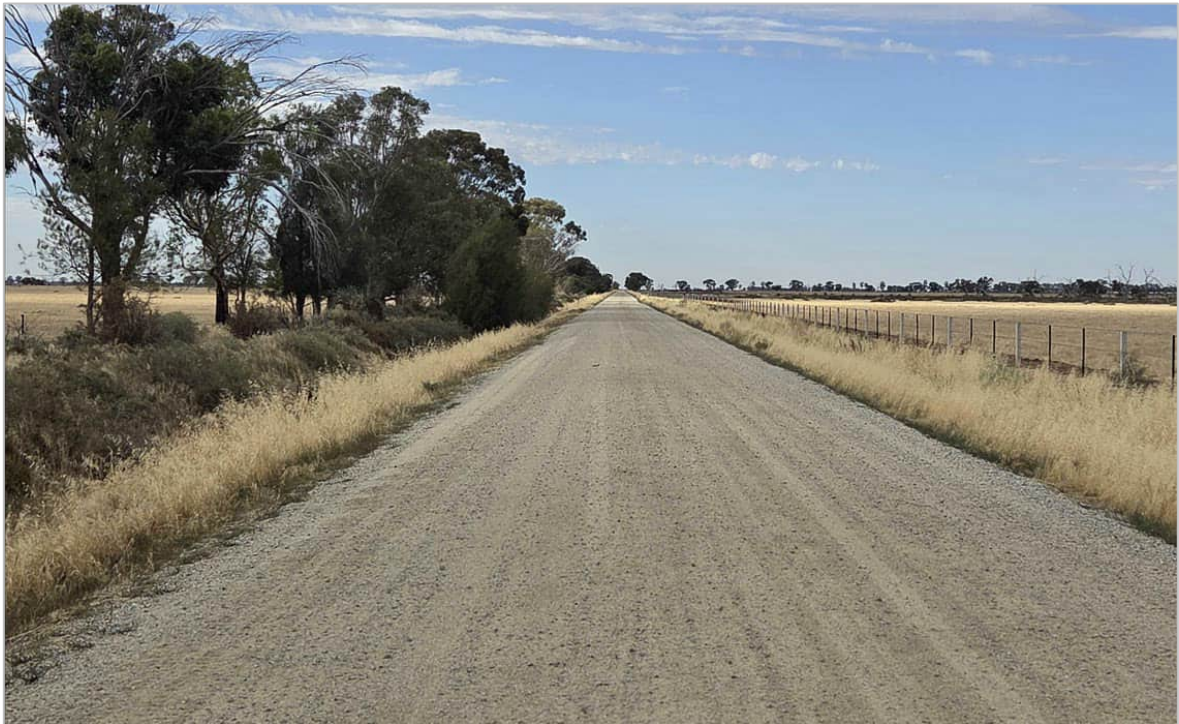
Figure 34: Typical All Weather (Gravel) Road – Mills Road
