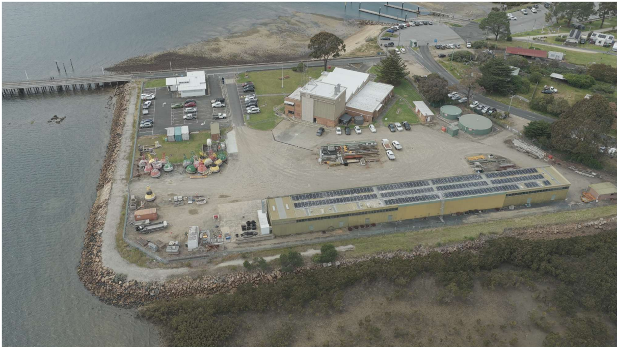
Figure 1: Stony Point Depot (Main Office)
