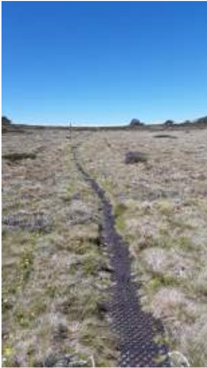
Image 1. Black matting track surface along a section of existing track, Bogong High Plains (December 2020), (Image credit: Louise Rodda)
