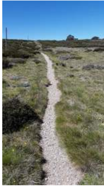
Image 2. River pebbles track surface along an existing track, Bogong High Plains (December 2020), (Image credit: Louise Rodda)
