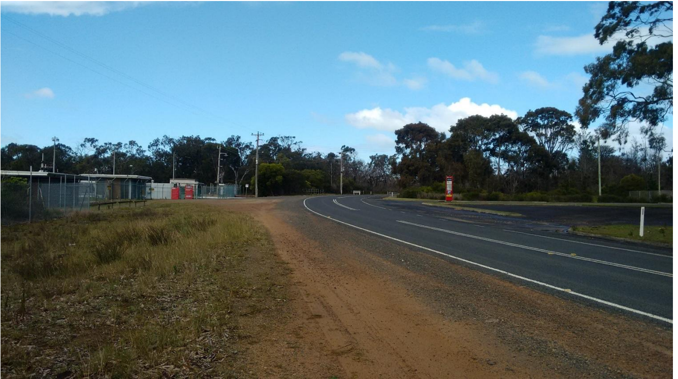
Figure 4.14 : Support buildings associated with the existing Crib Point Jetty
