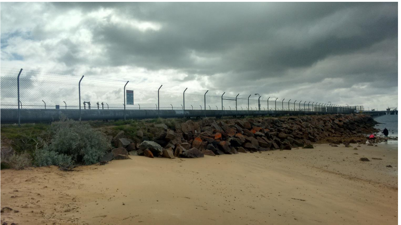
Figure 4.13 : Existing pipeline on the existing Crib Point Jetty
