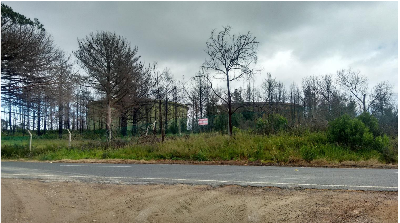
Figure 4.11 : Storage tanks associated with the former refinery
