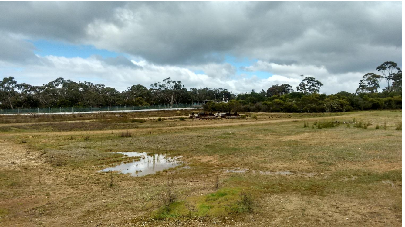
Figure 4.12 : Pipeline heading west from the existing Crib Point Jetty
