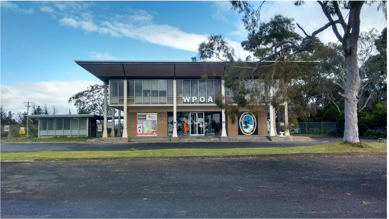
Figure 4.2 : Victorian Maritime Centre, Former BP building
