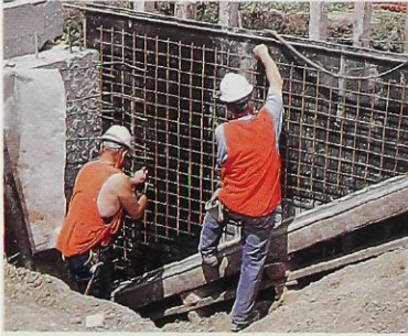
Improvements to the Calder Highway north-west of Melbourne.
