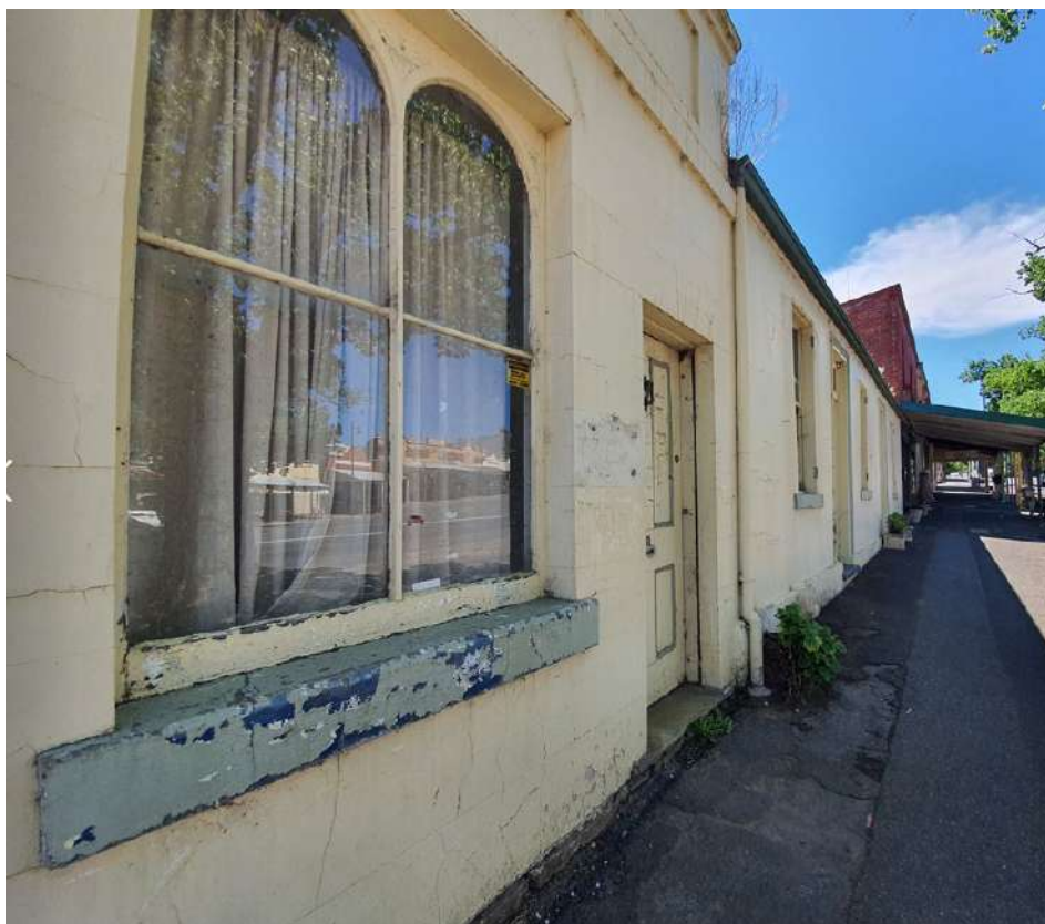
Figure 8. 1877 addition finished with ruled render (now overpainted) and decorative four-pane window. Note the ruled render has been applied across the entire street frontage. (Source: GML 2021)
