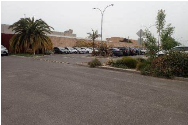
Figure 46. Garden areas at the east end of the carpark, contained within raised kerbing, facing southwest
