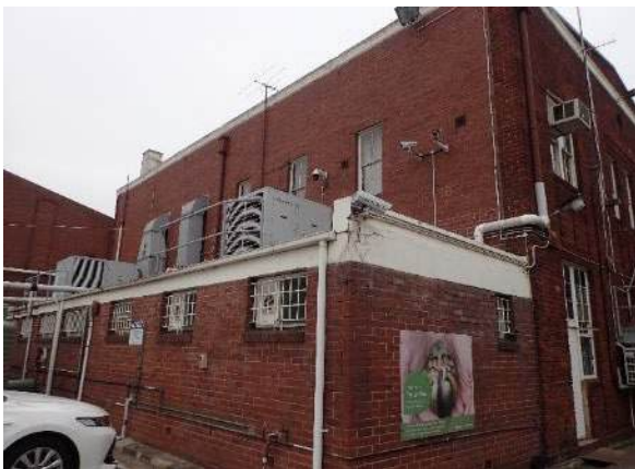
Figure 3-3 View of the Traffic and Revenue office building, facing northeast
