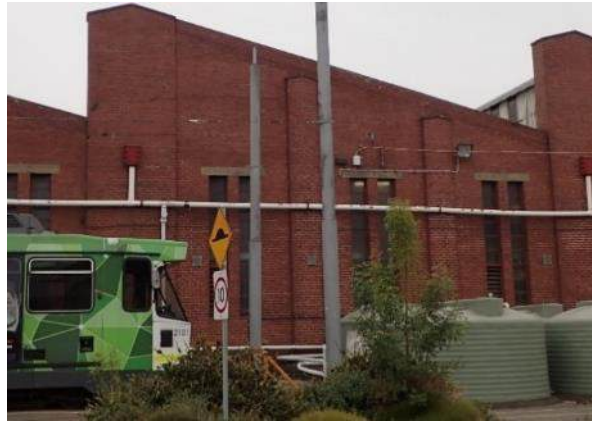
Figure 69. End of Roads 10 and 11 adjacent to the set of four tanks, facing north
