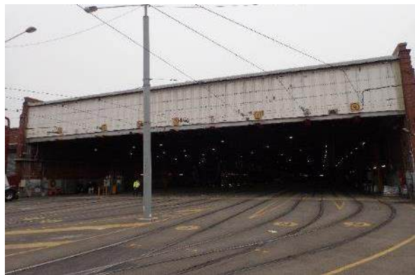
Figure 73. View across Roads 2 to 9 towards the tram shed, facing northeast
