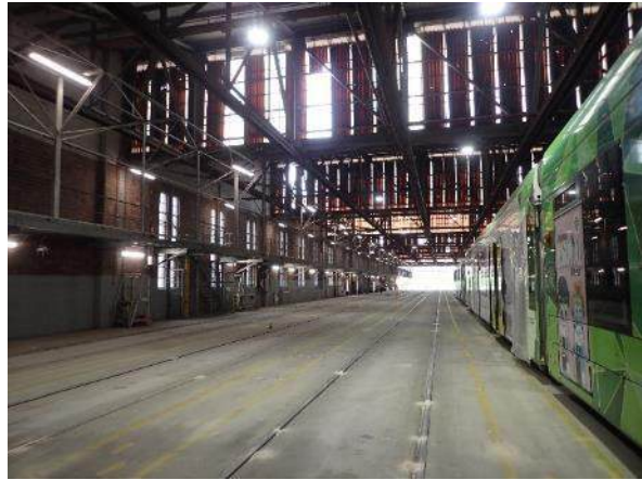
Figure 75. View of Roads 6 to 9 inside the tram shed building, facing west
