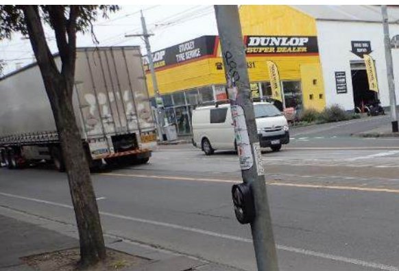
Figure 66. View of the roadway in the location of the original cable tram car entryway, facing northeast
