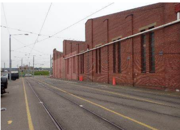
Figure 3-14 Roads 10 and 11 adjacent to the south face of the tram shed, facing west
