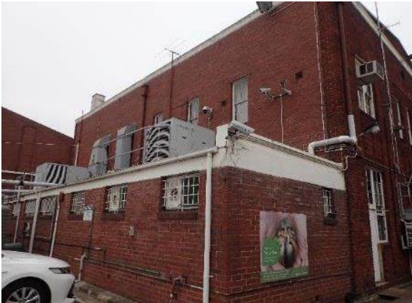
Figure 50. View of the Traffic and Revenue office building, facing northeast
