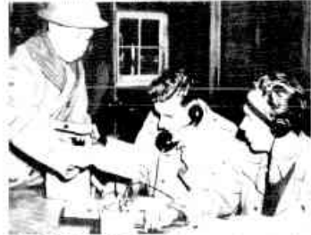
FIELD TELEPHONE and wireless operators at work.
