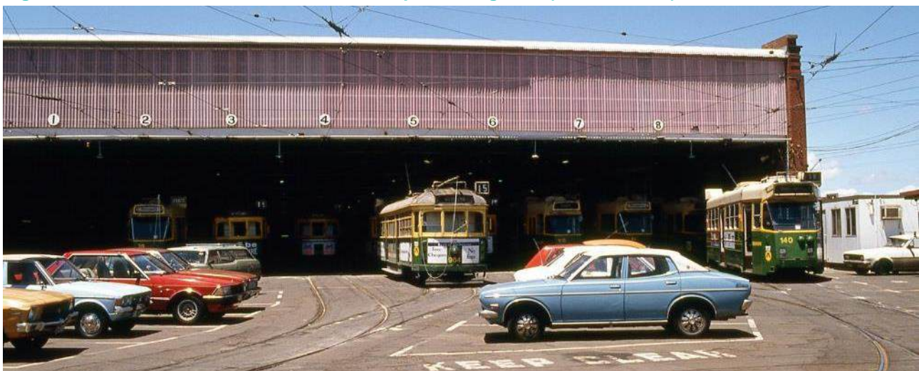
Figure 43. Rear of the Brunswick Tram Depot, facing east (Dunedoo 1989)
