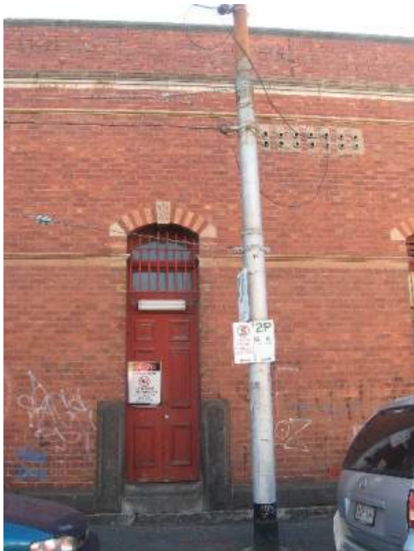
Brunswick cable tram engine house substation entrance
