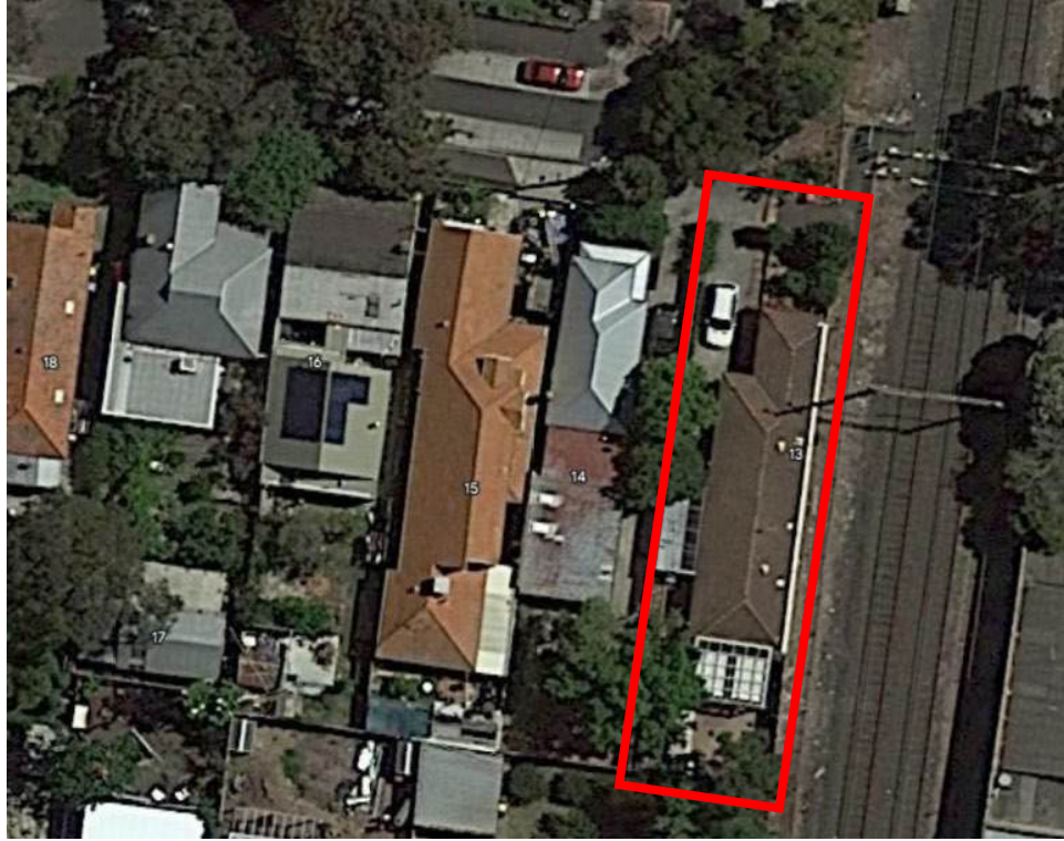
Figure 1: Demonstrating the footprint of the domestic dwelling of 13 Orient Grove, in red, oriented north, (Nearmap)
