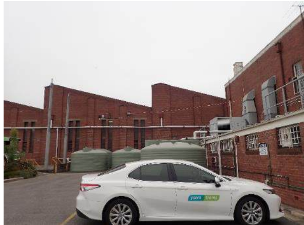
Figure 57. Tanks behind the Traffic and Revenue office building and beside the tram shed, facing north
