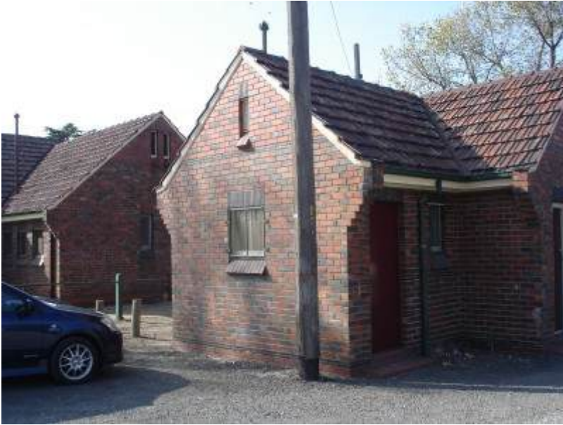
royal park toilet block pavilion apr07 jmb
