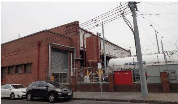
Figure 3-23 Roller door leading into the former wheel grinding workshop, facing southeast
