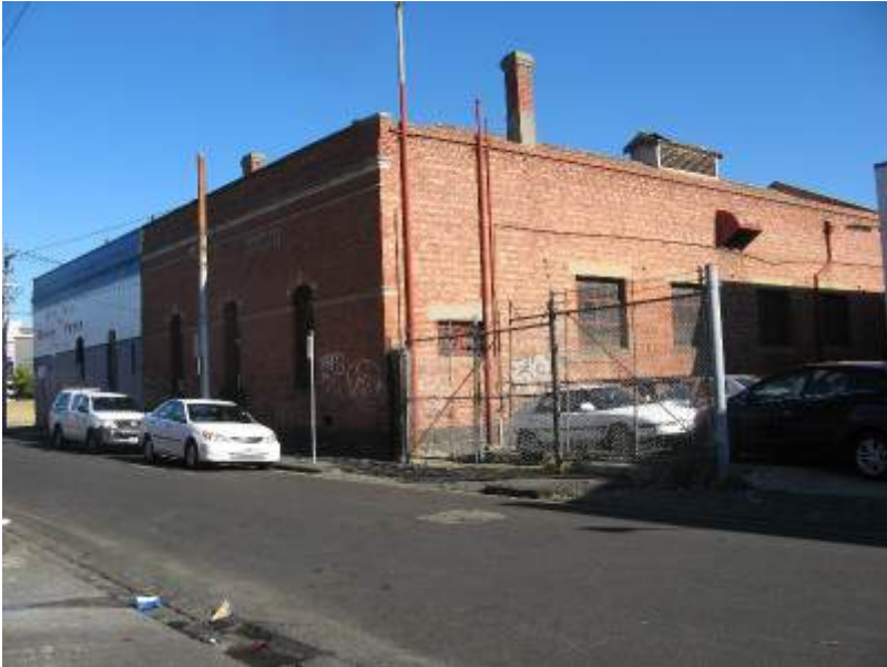
Brunswick cable tram engine house - substation
