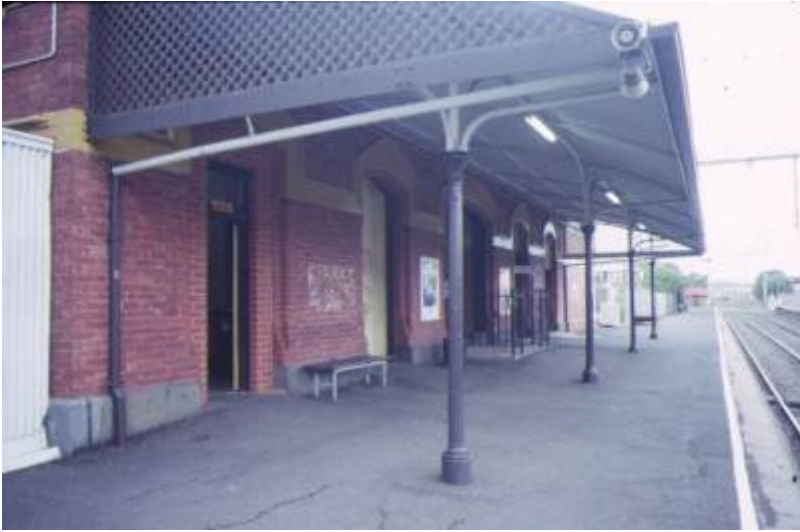
1 upfield railway line precinct parkville brunswick road brunswick platform
