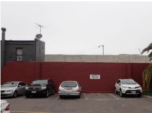
Figure 58. Carparking and brick wall along south boundary of the property, facing south
