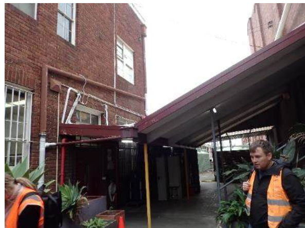
Figure 3-4 View of Traffic and Revenue office building and undercroft, facing southwest
