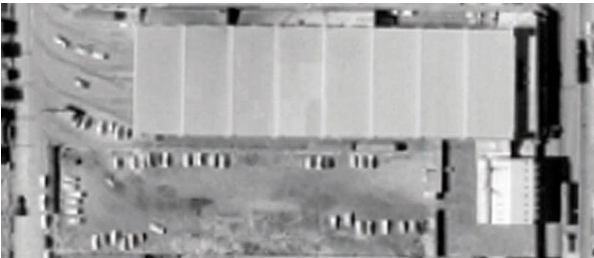
Figure 21. 1968 aerial imagery of the Brunswick Tram Depot site showing the 1936 Brunswick Tram Depot buildings, with a car parking area behind the Traffic and Revenue building (DELWP 1968)
