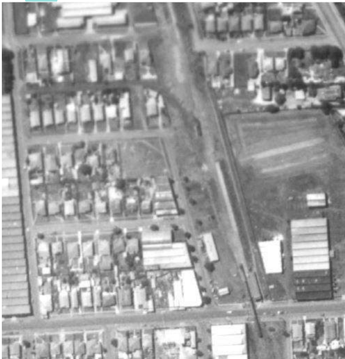
Figure 34: 1956 aerial photograph of Gaffney street intersection showing sidings along the western rail reserve, north of Gaffney Street. A structure is evidence alongside the sidings, east of Mantell Street. North is at top. (Bell and Moreland Level Crossing Removal Project, Heritage Assessment 2020).
