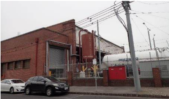
Figure 76. Roller door leading into the former wheel grinding workshop, facing southeast
