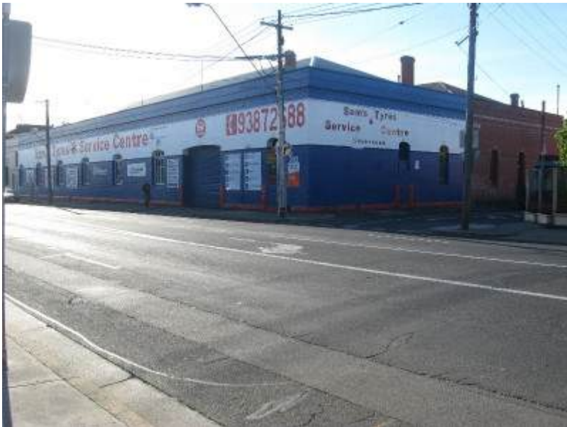
Brunswick cable tram engine house
