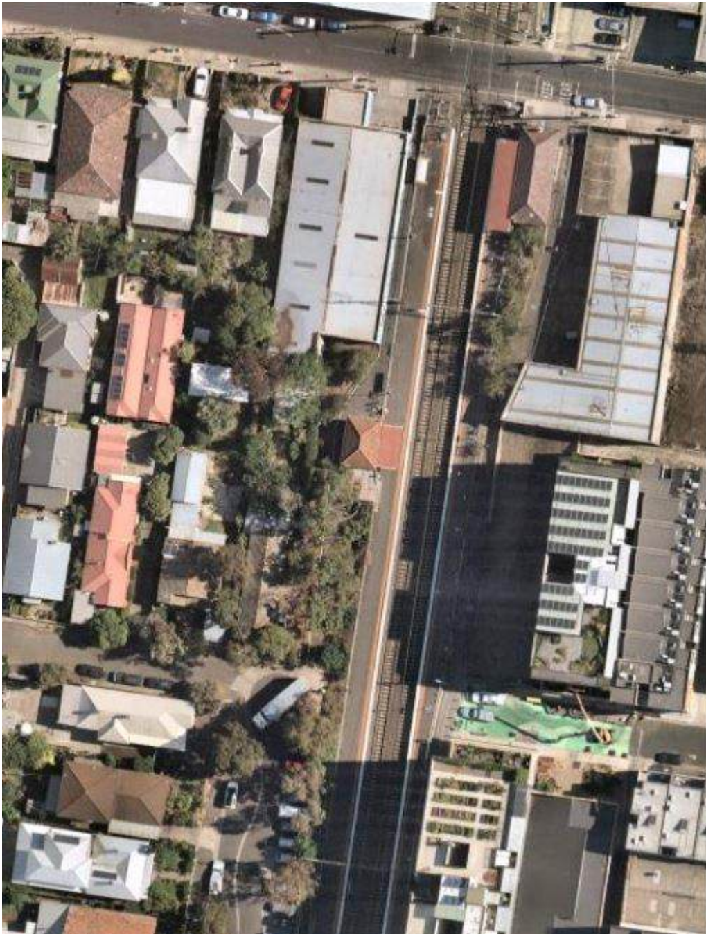
Figure 11: Current aerial photograph of the Albion Street intersection showing Anstey Station partially overlaying the footprint of the former gate-house at south-east of Albion Street. North is at top.
