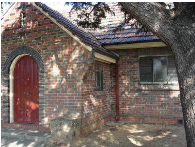
royal park pavilion front entrance detail apr07 jmb
