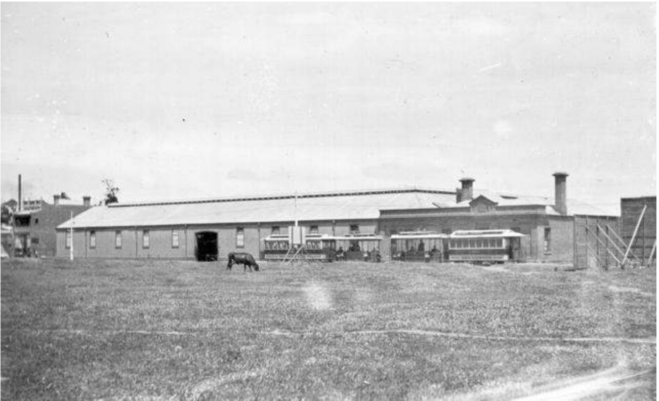
Figure 7. Undated early photograph of the Brunswick tram shed (left) and office building (right), with a tram car out the front, facing southwest across Sydney Road (Coburg Historical Society n.d.)
