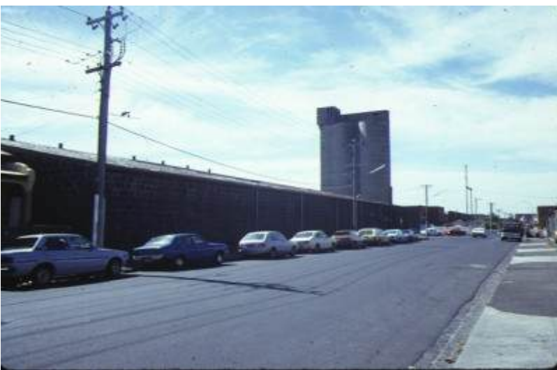
former melvilles grainstore colebrook street brunswick side elevation building 2
