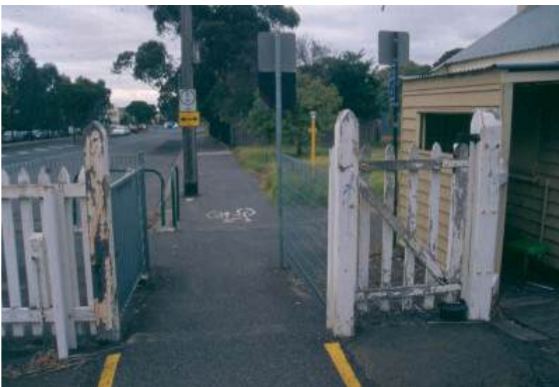
Upfield Railway Line Precinct Park Street Brunswick May 2006
