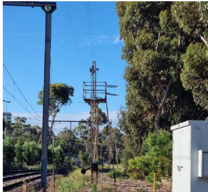
Figure 8: Extant semaphore at Park Street level crossing, view facing west
