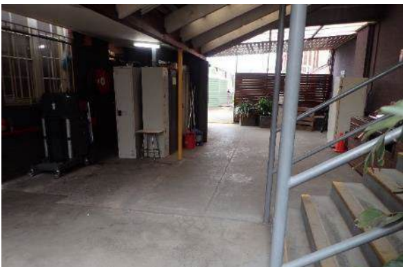
Figure 3-8 View of undercroft between the Traffic and Revenue office and tram shed, facing west
