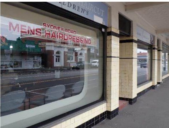
Figure 82. View of the shopfronts attached to the tram shed, facing northwest
