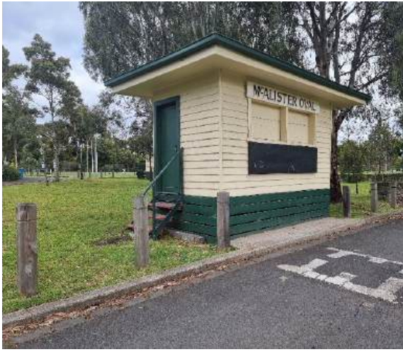
Figure 1: McAlister Oval sports pavilion, view facing north west
