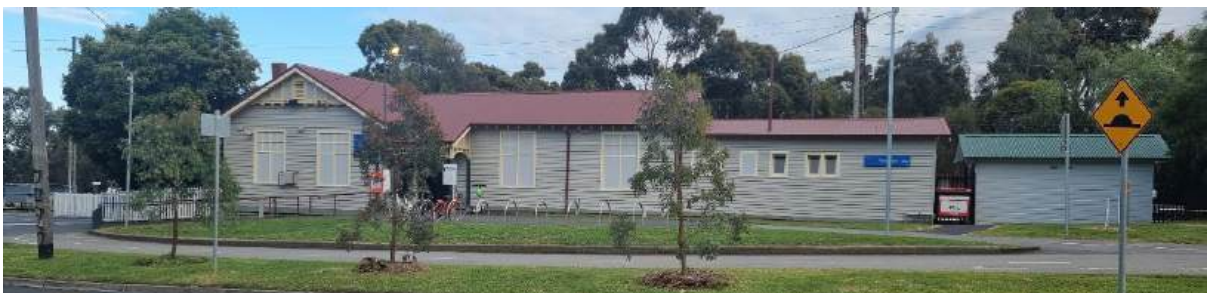
Figure 4: Royal Park Railway Station, view facing north
