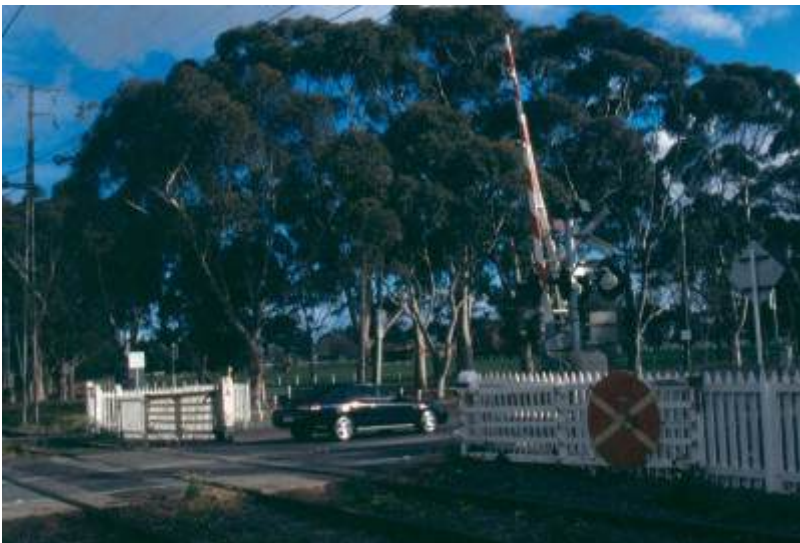
Brunswick Road Level Crossing Gates
