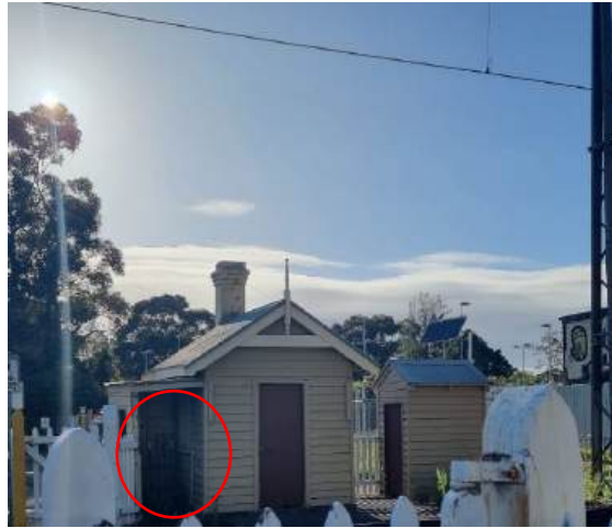
Figure 7: Extant signalling mechanism, indicated in red, view facing south
