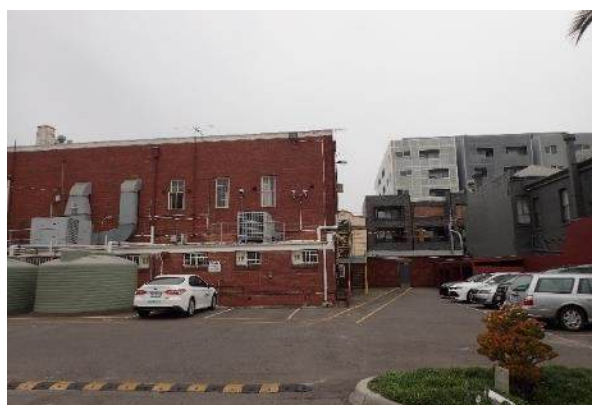
Figure 61. Rear of Traffic and Revenue office building, Sydney Road wall, and carparking, facing east
