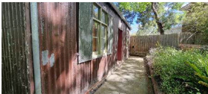
Figure 12: Rear face, non-renovated side of Walmsley House, view north
