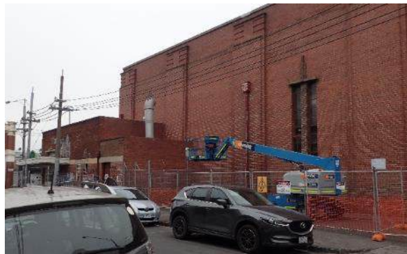
Figure 79. View of the substation and shopfront attached to the tram shed (note cherry picker), facing southeast
