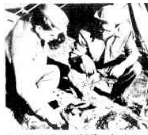
CHECKING AND MENDING a break in the field wire for telegraphing.
