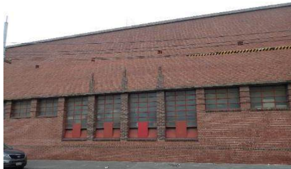
Figure 77. Detail of the workshops attached to the tram shed along Peveril Street, facing south
