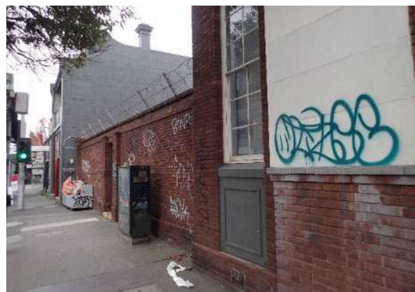
Figure 3-6 View of wall between the Traffic and Revenue office building and the adjacent building, facing southwest
