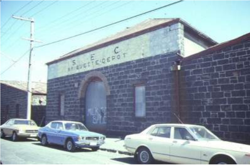
former melvilles grainstore colebrook street brunswick entrance
