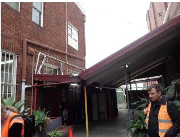
Figure 52. View of Traffic and Revenue office building and undercroft, facing southwest
