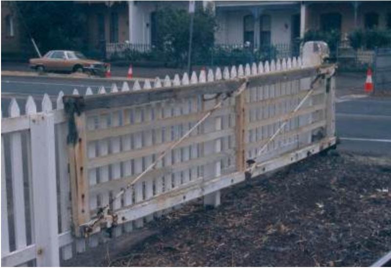
Upfield Railway Line Precinct Park Street Brunswick May 2006
