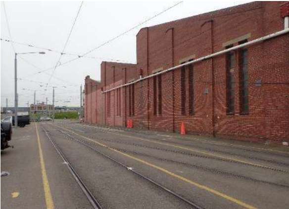
Figure 68. Roads 10 and 11 adjacent to the south face of the tram shed, facing west
