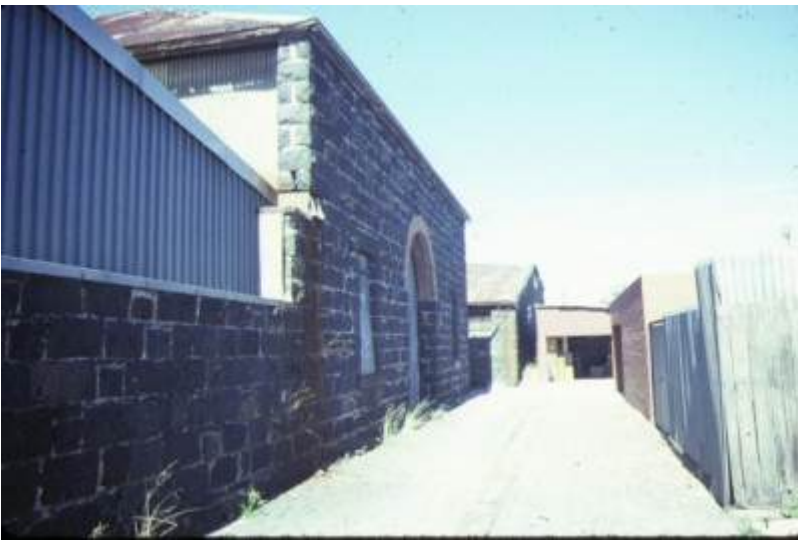
former melvilles grainstore colebrook street brunswick rear of buildings 3 & 4
