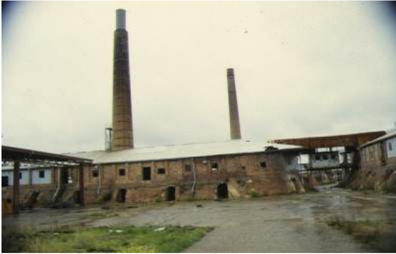
Former Ferry Terra Cotta & Enamelled Brickworks Office Albert Street Brunswick Kiln 1997
