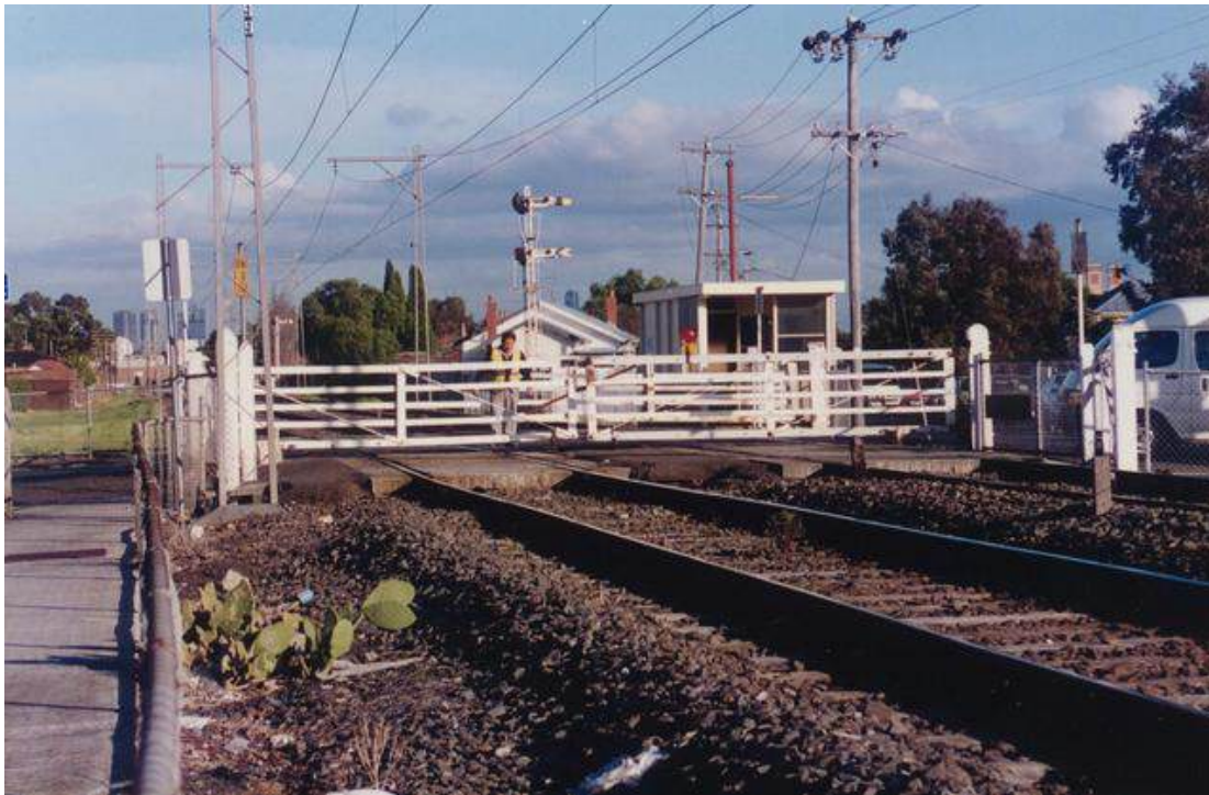
Figure 30: 1992 photo of hand-gates at O'Heas Street, facing south. Gatekeepers cabin visible in background. (Trove website, 10/06/2020).
