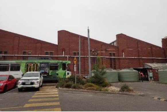
Figure 62. Set of four tanks at the end of Roads 10 and 11 adjacent to the tram shed and carpark garden, facing north
