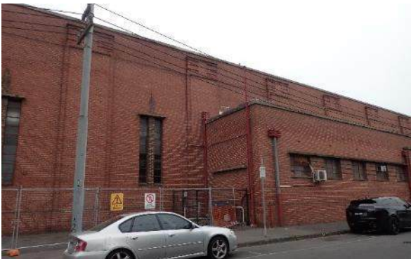
Figure 78. View of the east end of the workshops attached to the tram shed, facing southwest
