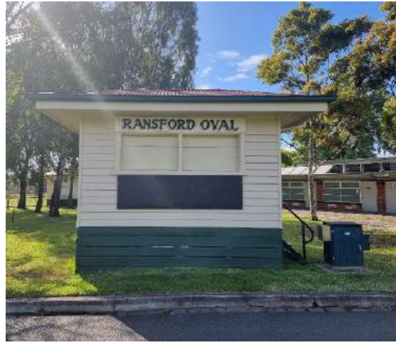
Figure 2: Ransford Oval sports pavilion, view facing west
