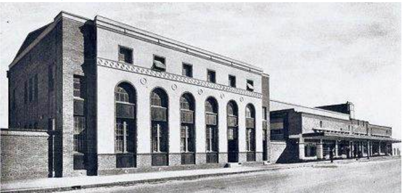
Figure 17. Official MMTB photograph (1936) of the newly constructed depot, prior to the installation of the tramway's overhead powerlines (Jones 2014)
