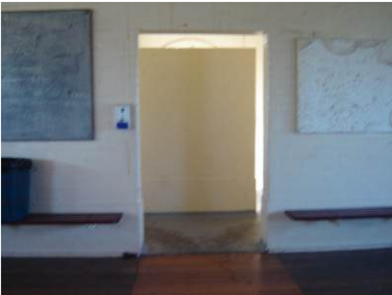
poplar oval pavilion interior exit jun07 jmb
