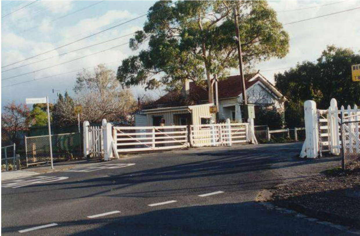
Figure 21: 1998 photo of hand-gates at Reynard Street with gatekeepers cabin visible. (Trove website, 10/06/2020).
