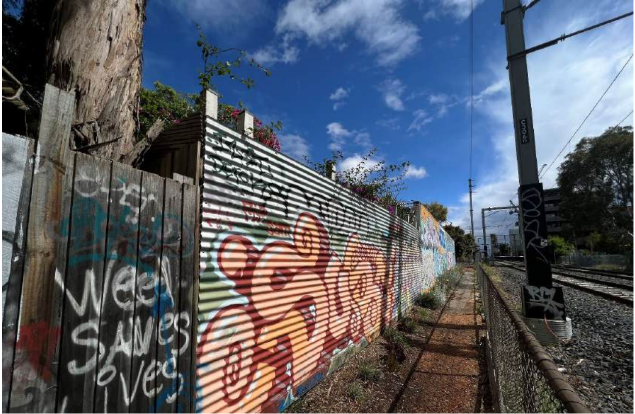
Figure 3: Eastern side fence of 13 Orient Grove adjacent to the Upfield railway line corridor, view facing north
