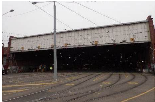
Figure 3-19 View across Roads 2 to 9 towards the tram shed, facing northeast
