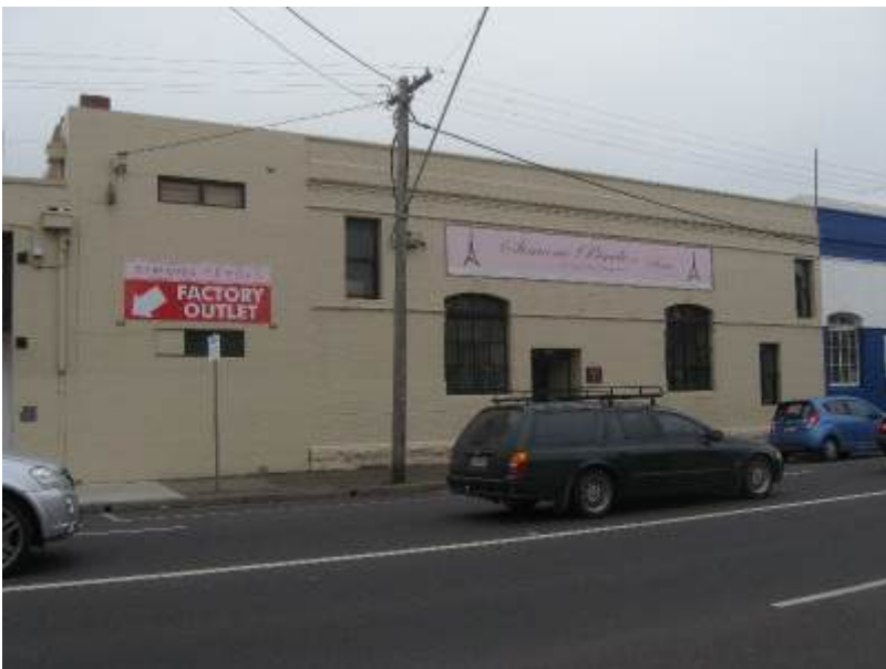
Brunswick cable tram engine house 261-63 Brunswick Road
