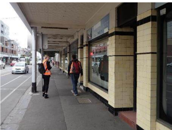
Figure 84. View of the shopfronts attached to the tram shed, facing south
