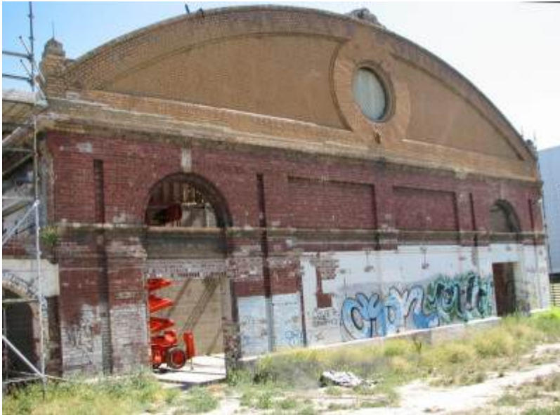
FORMER BRUNSWICK GAS & COKE COMPANY RETORT HOUSE SOHE 2008
