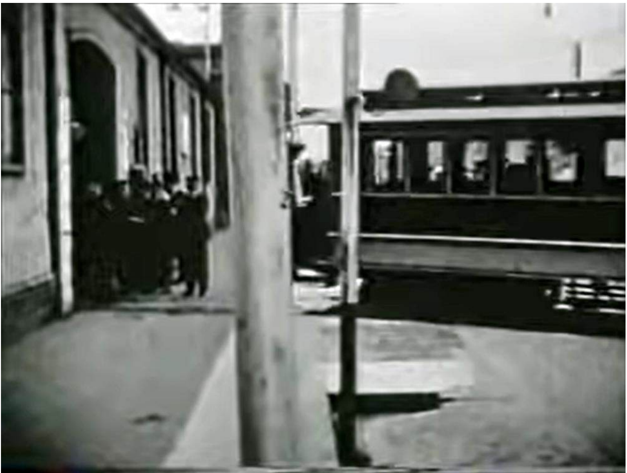
Figure 14. Cable tram being moved from Sydney Road into the Brunswick tram shed (Govett 1933-1939)
