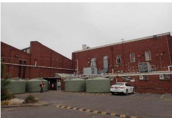
Figure 60. Tanks adjacent to tram shed and the Traffic and Revenue office, and carparking next to office, facing northeast
