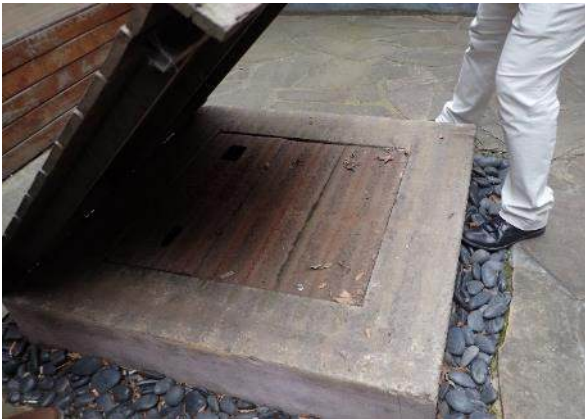
Figure 3-10 Close up of well with metal covering under timber seating, facing west
