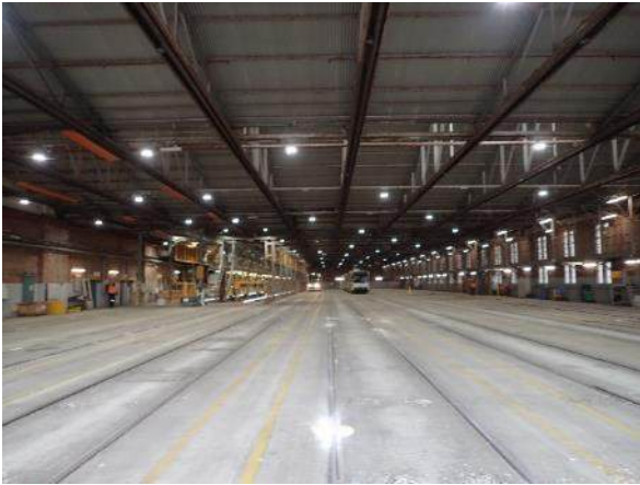
Figure 74. View of Roads 2 to 9 inside the tram shed building, facing east
