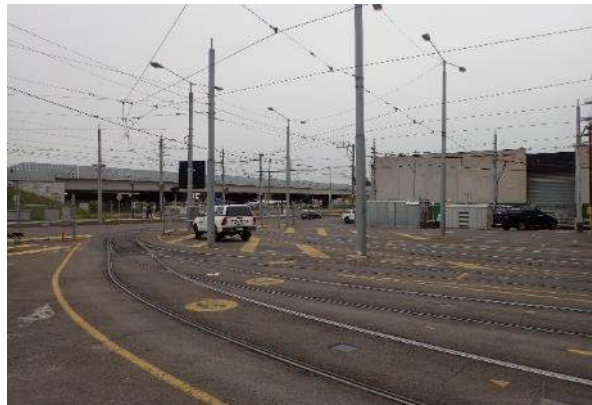
Figure 71. Roads 2 to 9 and associated track fans near Cameron Street, facing north
