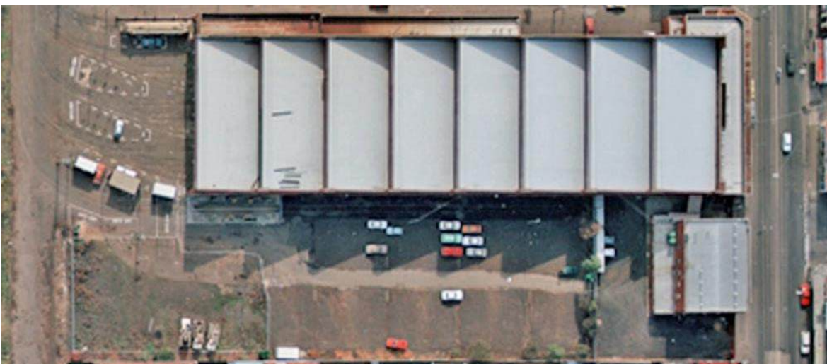
Figure 22. 1988 colour aerial imagery of the Brunswick Tram Depot site showing the 1936 Brunswick Tram Depot buildings (DELWP 1988)
