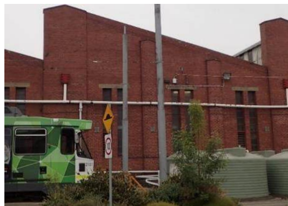
Figure 3-15 End of Roads 10 and 11 adjacent to the set of four tanks, facing north
