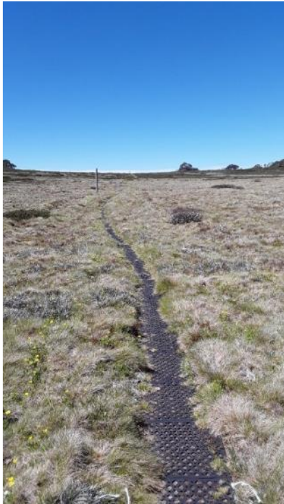
Image 2. Black matting track surface along a section of existing track, Bogong High Plains (December 2020), (Image credit: Louise Rodda)
