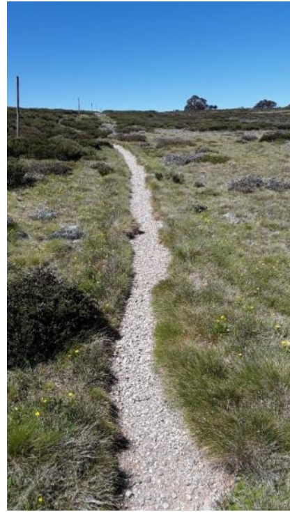
Image 3. River pebbles track surface along an existing track, Bogong High Plains (December 2020), (Image credit: Louise Rodda)
