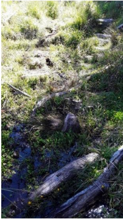
Image 10. Failed section of log track with pugging along Westons Spur Track (December 2020), (Image credit: Matthew Hatton)
