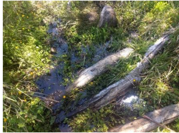
Image 11. Displaced, sunken logs as part of a log crossing on Westons Spur Track (December 2020), (Image credit: Matthew Hatton)
