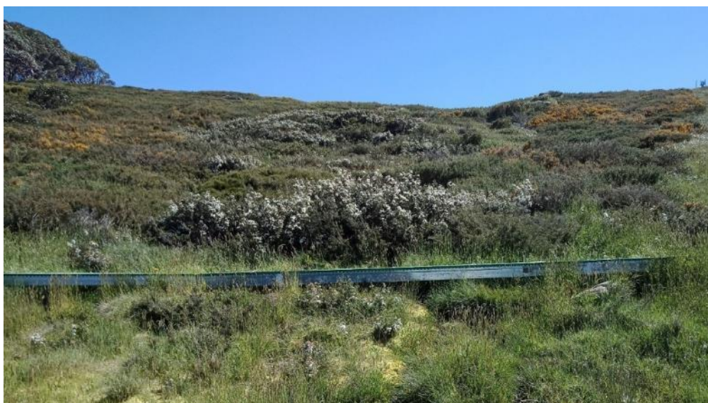
Image 104. Example of steel bridging over a drainage line intersecting Pretty Valley Road within the Falls Creek Alpine Resort boundary (December 2020), (Image credit: Louise Rodda)
