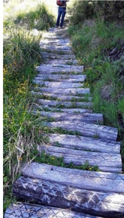
Image 9. Parallel logs laid along contour lines used to stabilise part of Westons Spur Track (December 2020), (Image credit: Matthew Hatton)
