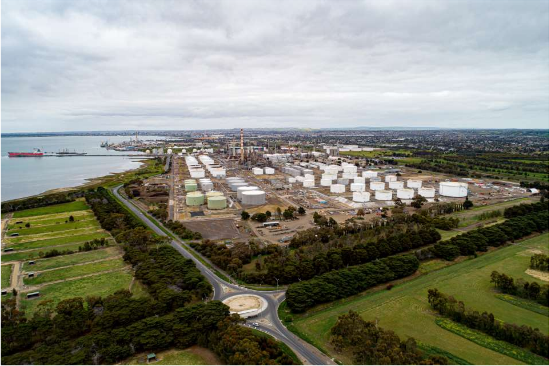
Photograph 3: View south over Geelong Refinery and Refinery Pier
