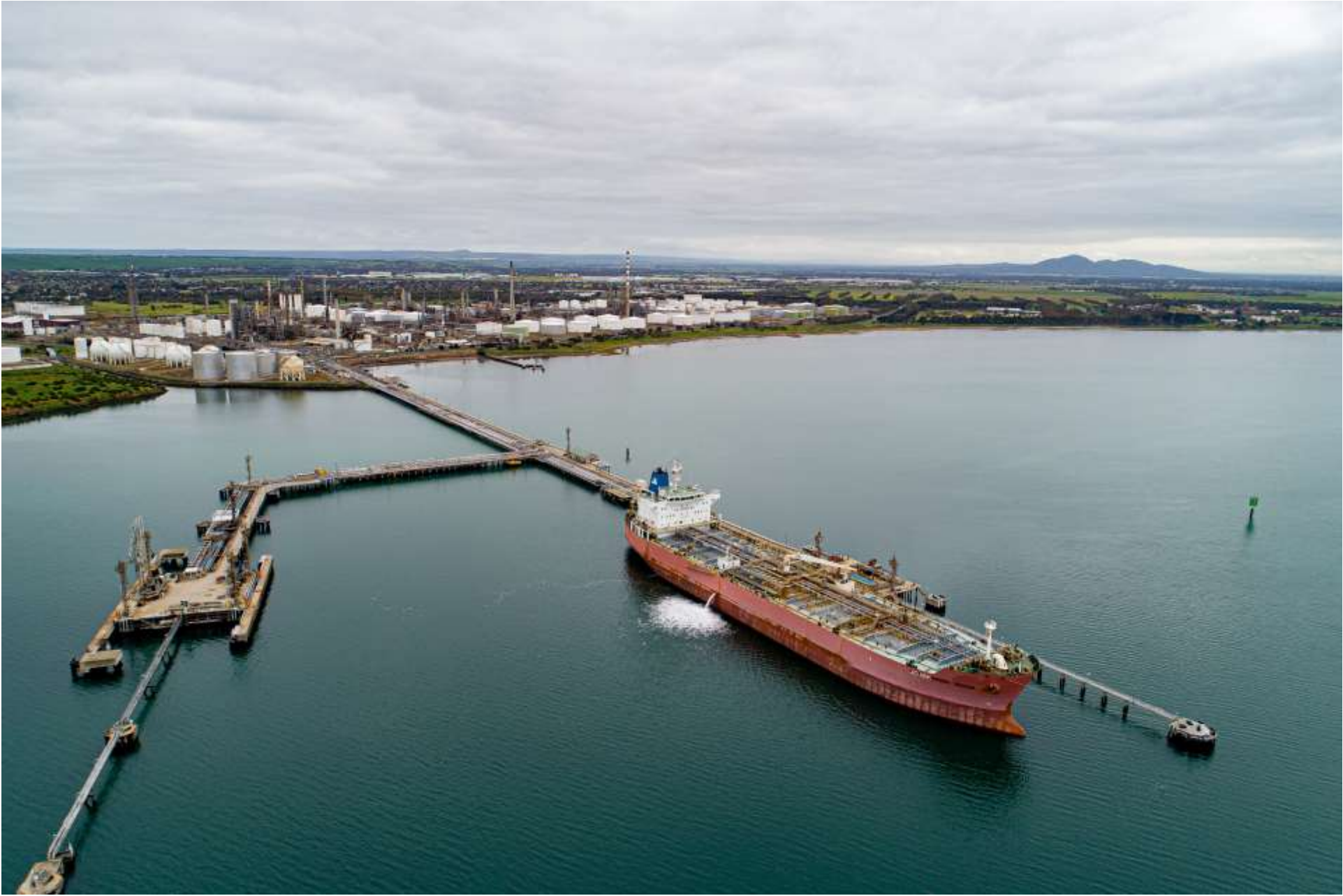
Photograph 1: View over Refinery Pier to the Geelong Refinery and north along the proposed pipeline corridor
