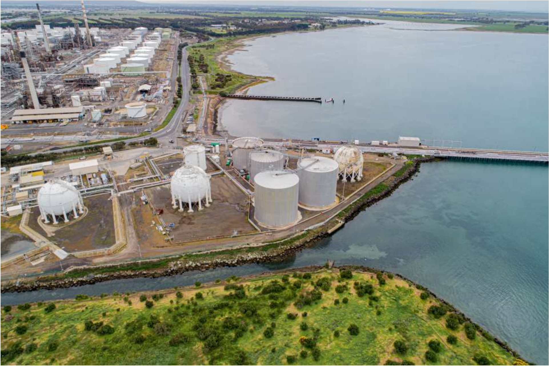
Photograph 2: View north over Geelong Refinery and along the proposed pipeline route.
