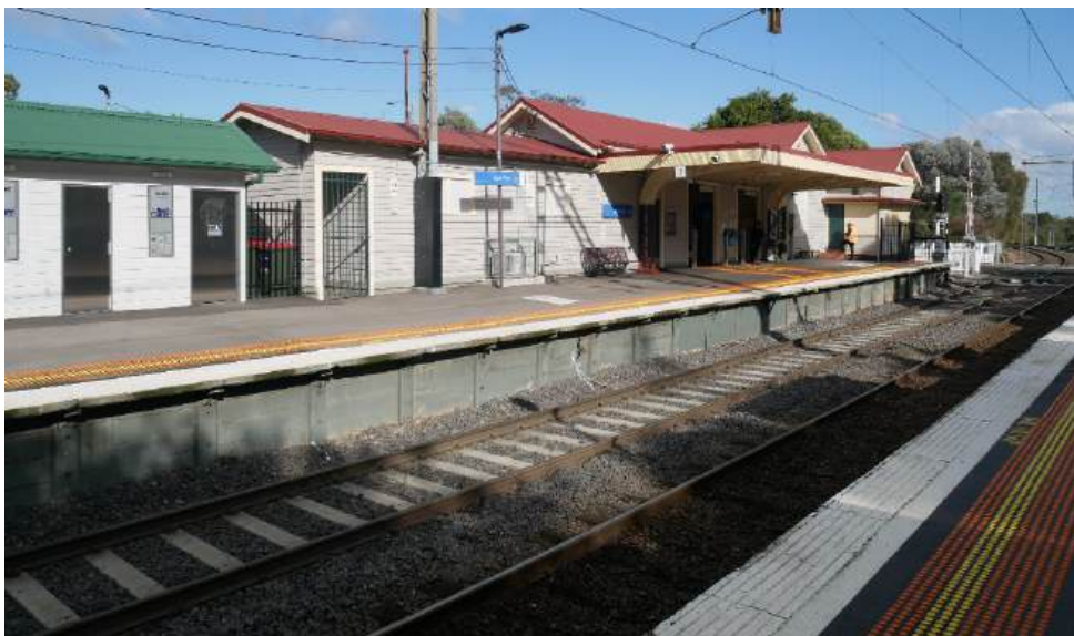
Figure 5. Image looking southwest from the down-side platform at Royal Park Station, showing station building with level crossing partially visible at right.
