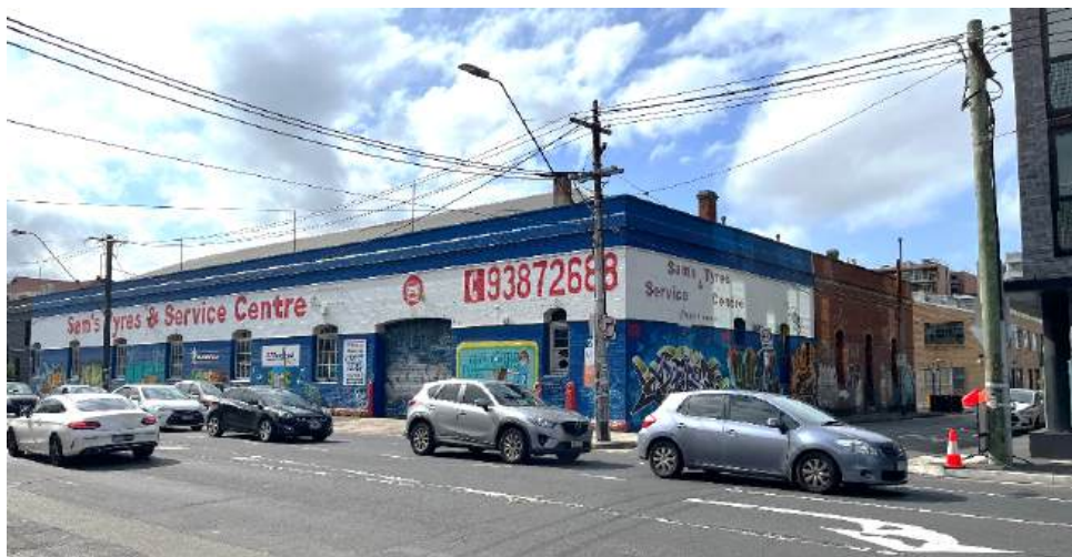
Figure 50. Looking northwest from the corner of Brunswick Road and Black Street to the Former Cable Tram Engine House & Tram Substation (VHR H2332).
