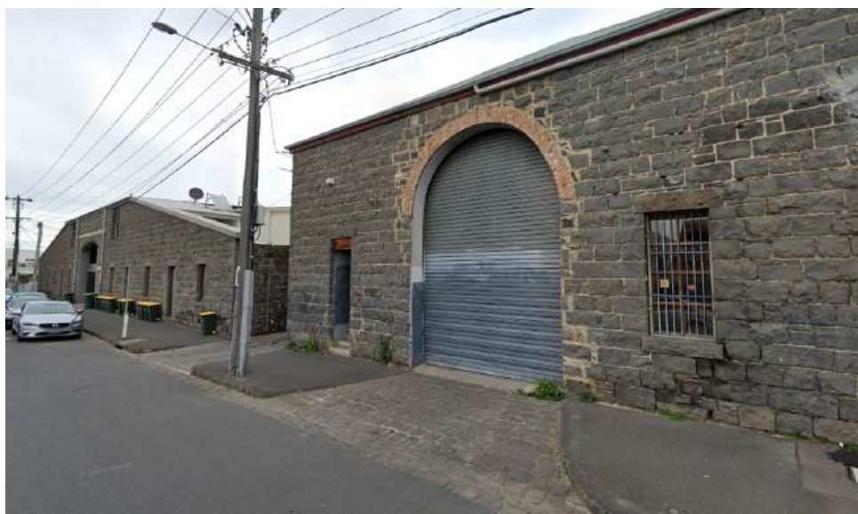
Figure 72. East elevation of part of the Former Melville’s Grain Store as viewed looking southwest along Colebrook Street. (Source: Google Streetview, image dated September 2022, accessed 16 November 2023)
