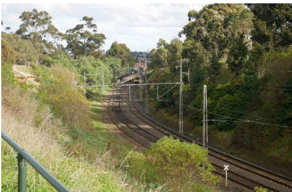
Figure 6. Image looking southwest from bicycle path above and east of railway line cutting. Royal Park Station partially visible at centre. Note grade change and steep batter.
