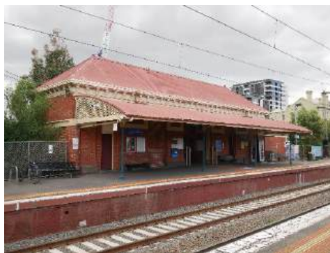
Figure 39 (left). Albert Street Gatekeepers Cabin and WC.
