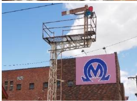
Figure 41 (left). Victoria Street Signal Box and WC.
