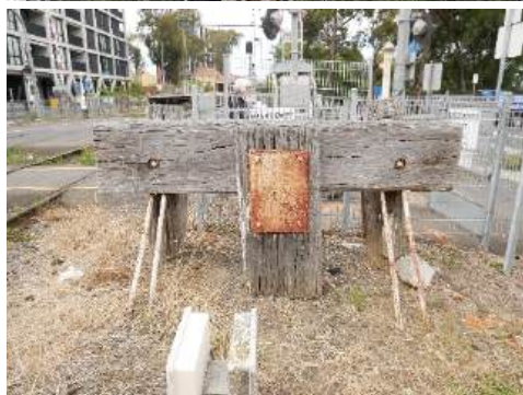
Figure 31 (left). Union Street gate posts.
