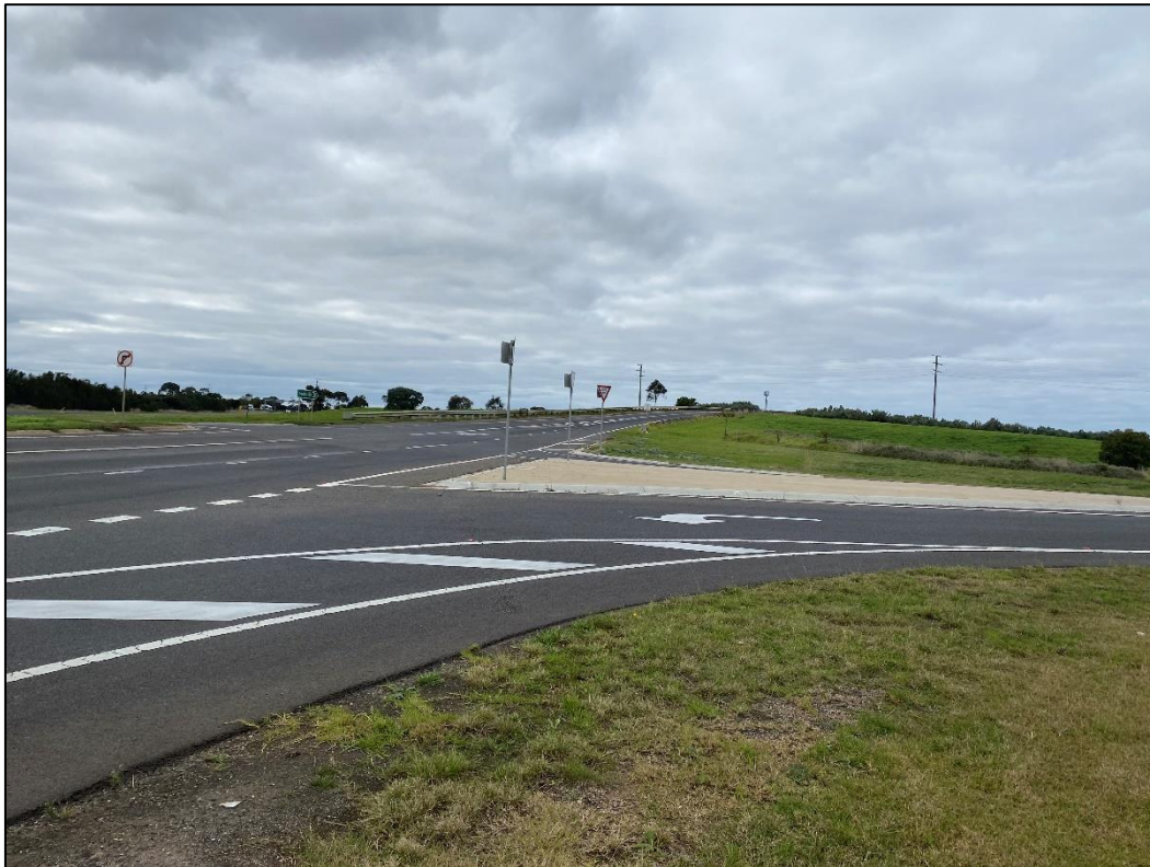
Princes Freeway/Little River Road interchange – from Geelong
