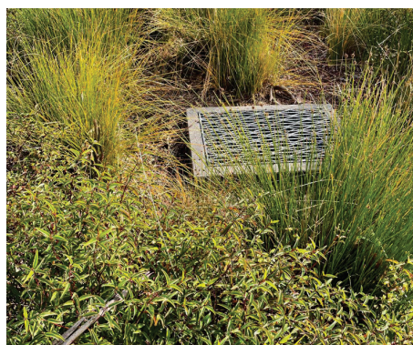
Rain gardens should be adjacent to large impervious areas like driveways and car parking areas.
