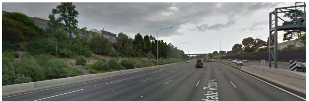
City Link provides good adjacent vegetation cover with a variety of groundcover, shrubs and trees, which are safely separated from traffic by a concrete barrier.
