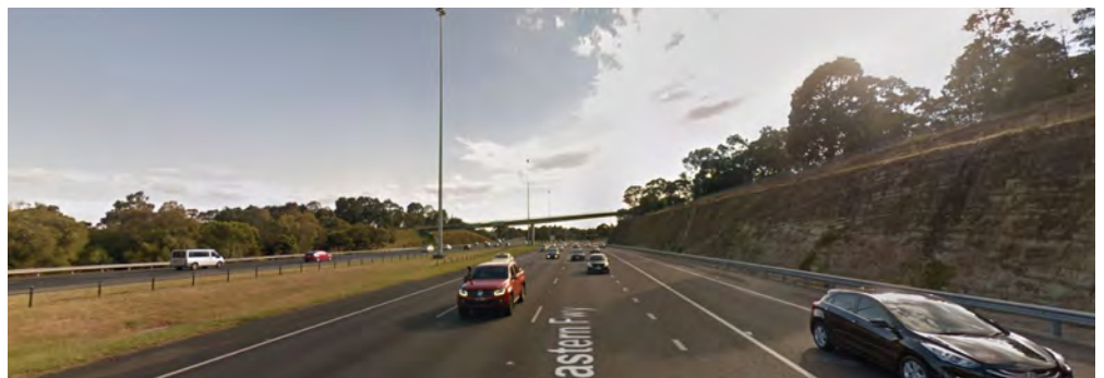
Eastern Freeway with grass verge in centre of highway separating direction of flow. Trees could be placed behind the flexible barrier.
