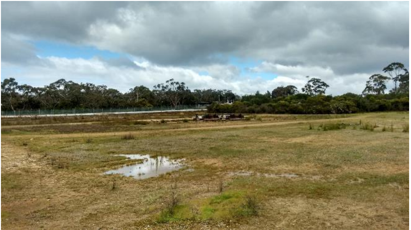
Figure 5: Pipeline Heading West from the Existing Crib Point Jetty (source: Jacobs)
