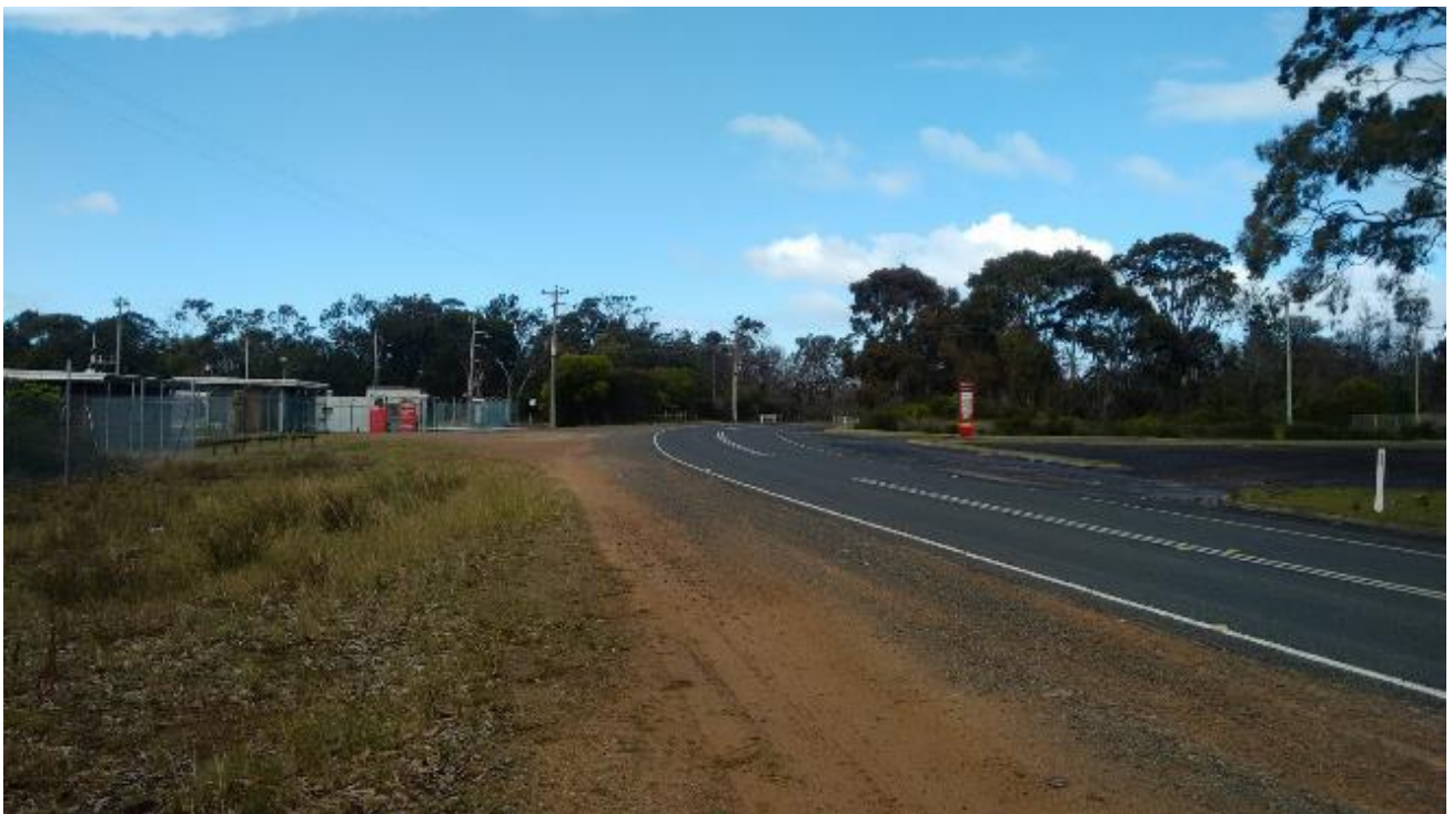
Figure 6: Support Buildings Associated with the Existing Crib Point Jetty (source: Jacobs)
