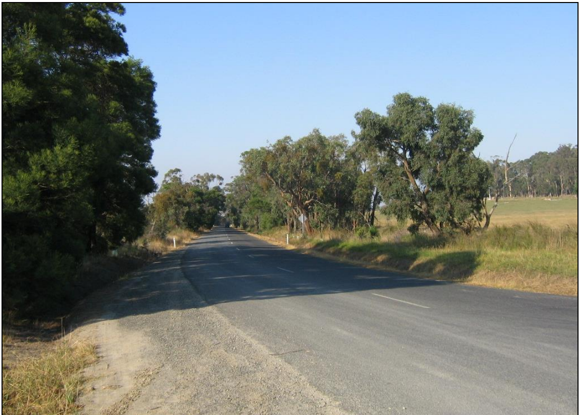
Figure 4 - Tonimbuk Road, sealed average condition
