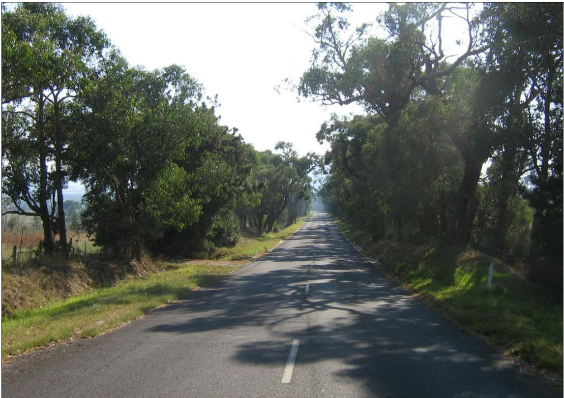
Figure 6 - North Garfield Road just north of its intersection with Princes Freeway, sealed average condition
