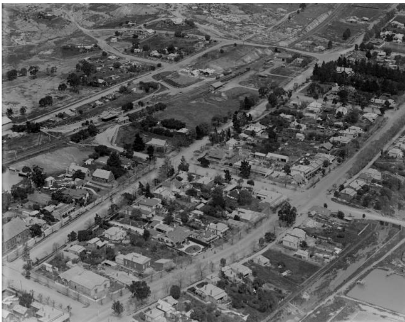
Figure 45. Aerial view of High Street and Pantom Street ca 1925-1940, Laurel Street is at the bottom left. (Source: Charles Daniel Pratt, State Library of Victoria)
