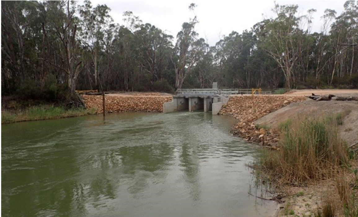
Figure 5: A containment bank constructed under The Living Murray at the Hattah Lakes, similar to those proposed for Burra
