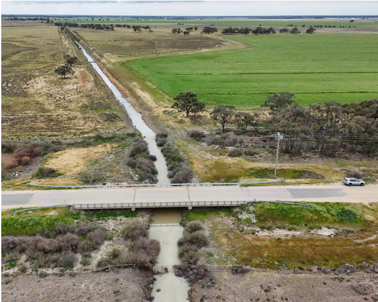
Figure 21- Old Echuca Road Main Drain
