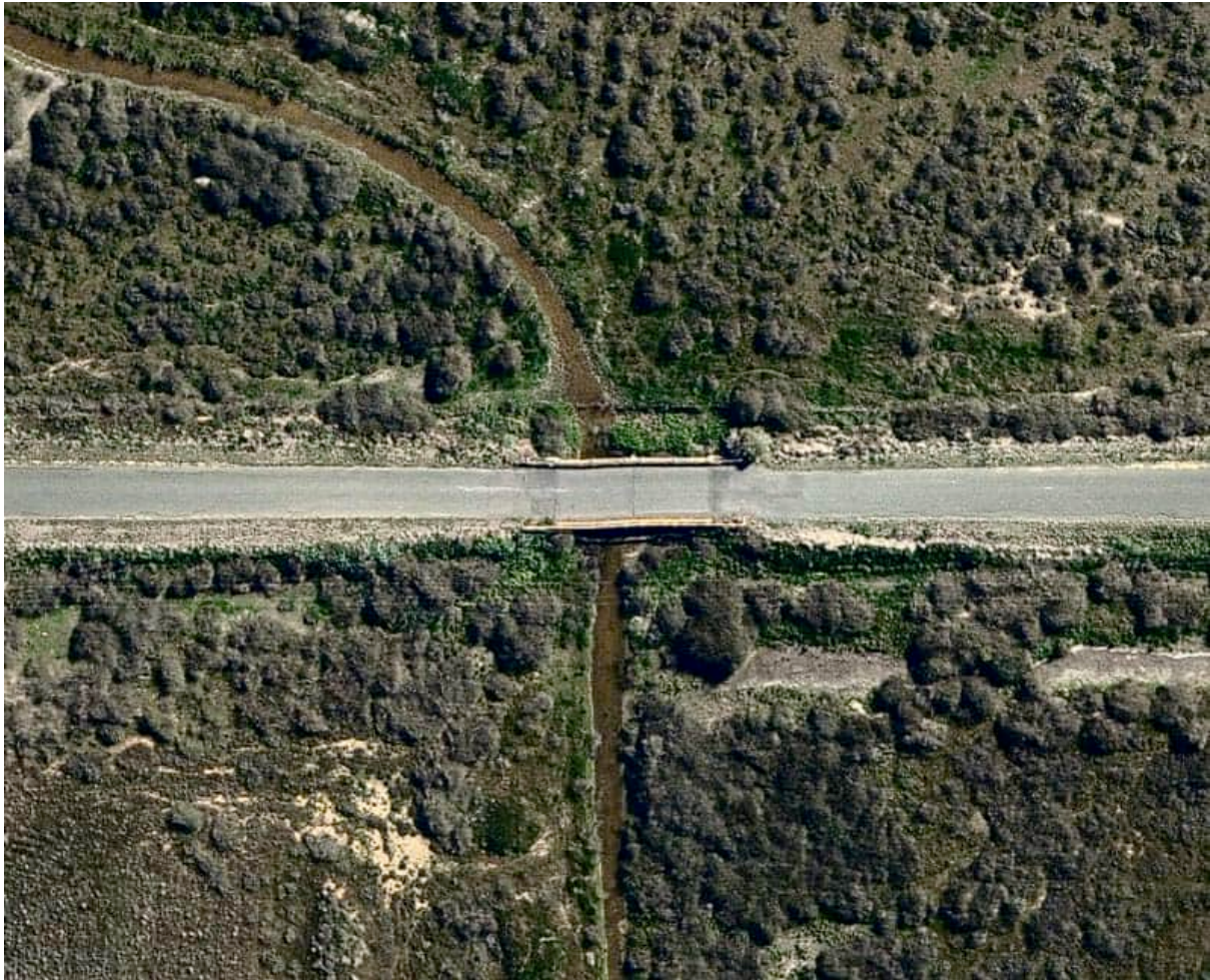
Figure 15- Calivil Creek Bridge on Macorna – Pyramid Road at Macorna
