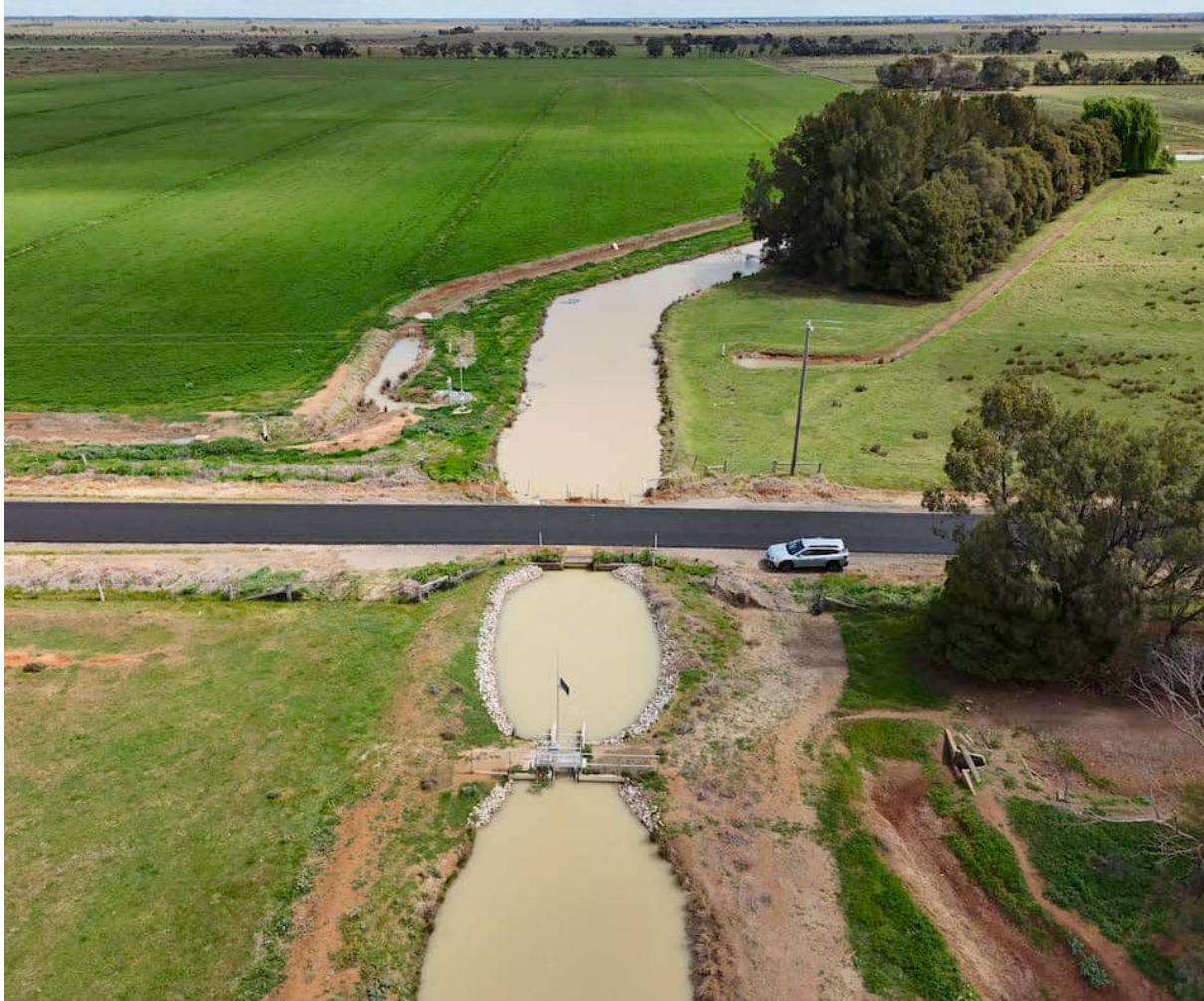
Figure 28- Macorna-Kerang Road drain/channel, Macorna
