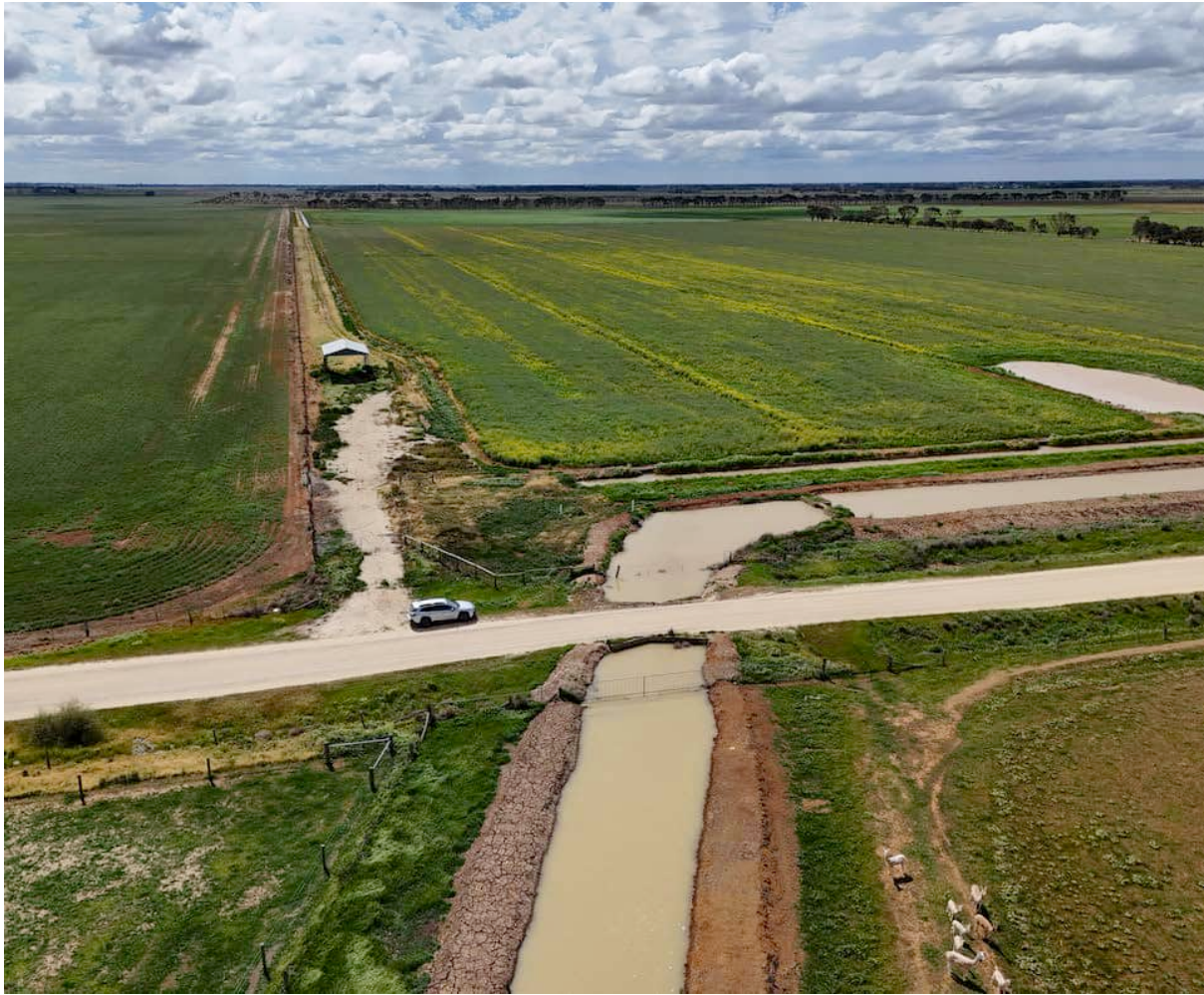
Figure 13- Macorna Road Bridge over Channel 10 / 1
