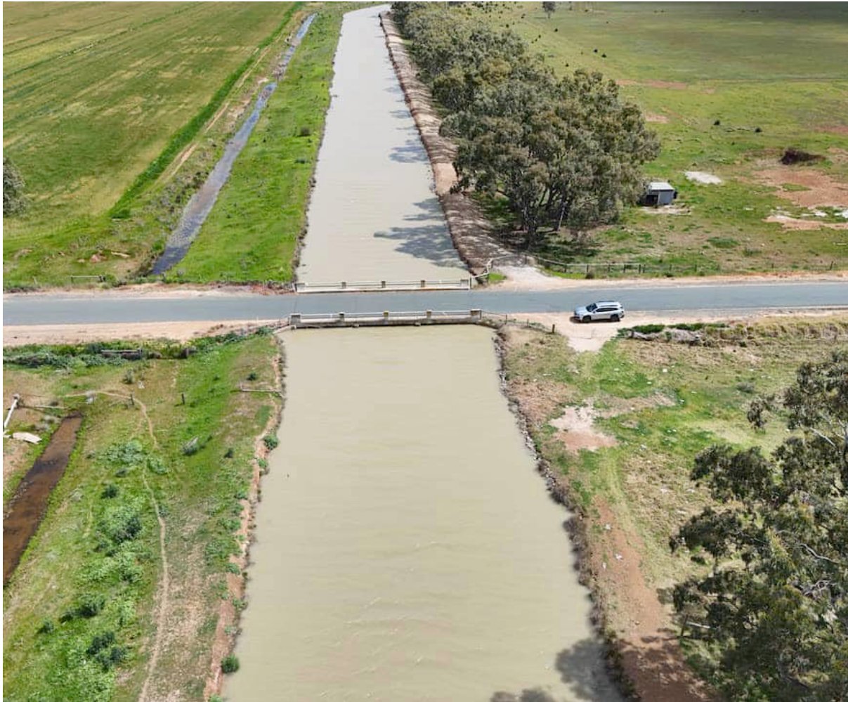
Figure 27- Macorna Channel, Macorna – Kerang Road
