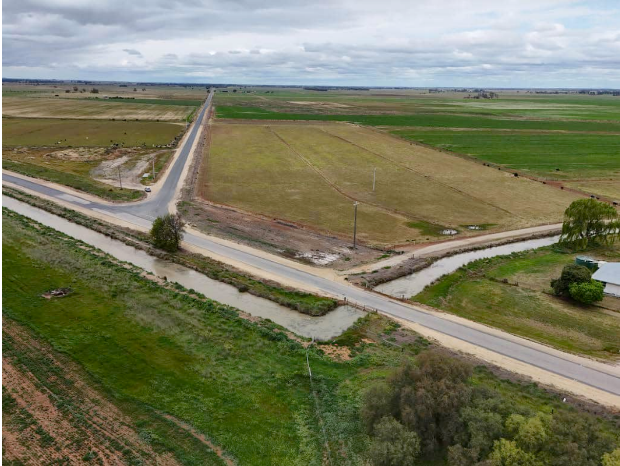
Figure 24- Leitchville -Macorna Road channel & Macorna- Kerang Road intersection
