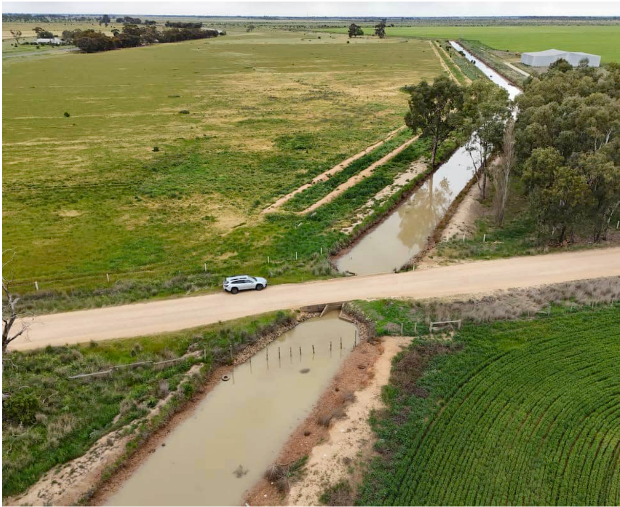
Figure 10- Macorna Road over Channel no. 12
