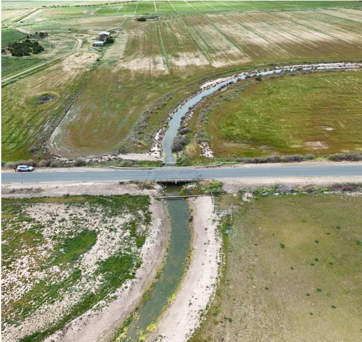
Figure 26- Macorna-Kerang Road drain/channel, Tragowel
