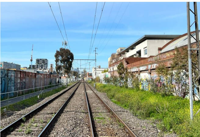
Figure 4 Planted vegetation along the rail corridor.
