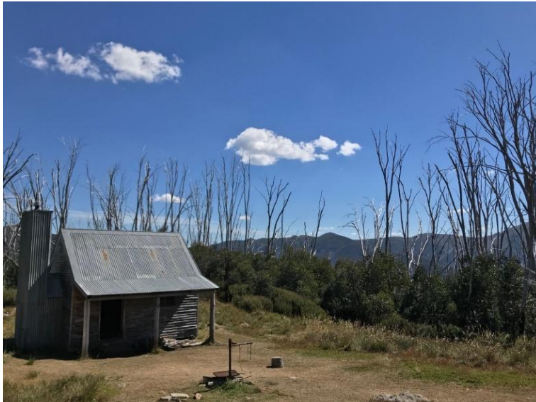
Figure 2.11 Westons Hut with picnic area in foreground. (Source: Parks Victoria)
