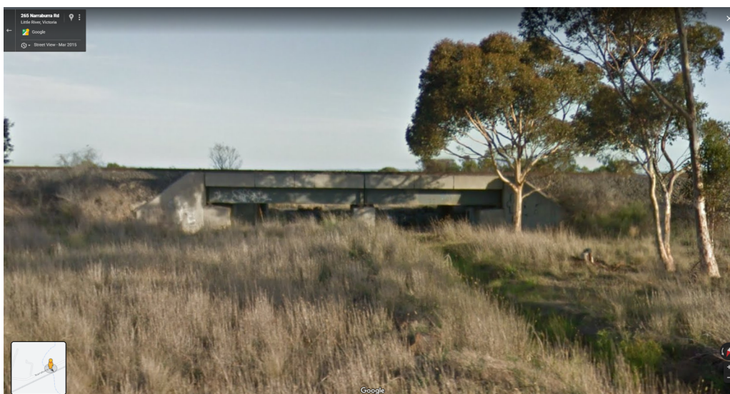
Figure 3– Photo of Ryan Swamp Drain Bridge – Source: Google Imagery
