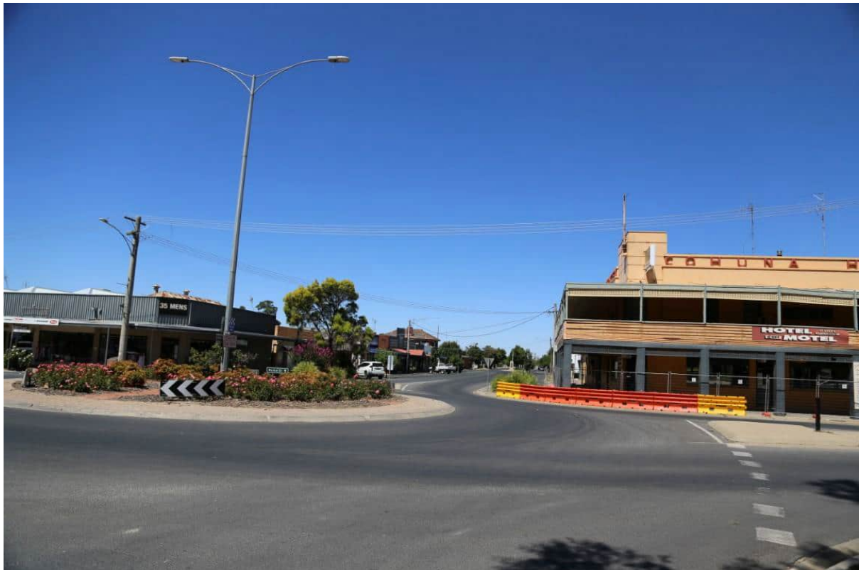
Figure 62 – VP1 – View towards Project Area.
