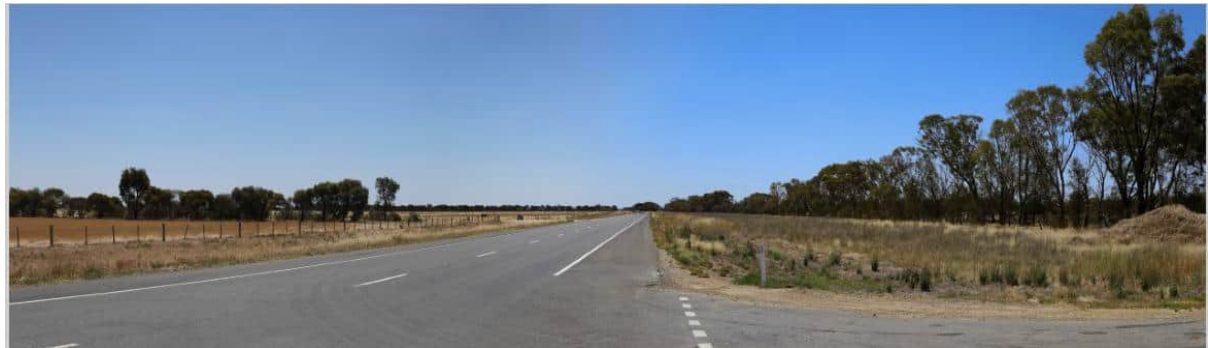
Figure 85 – VP5 –Existing view towards Project Area.
