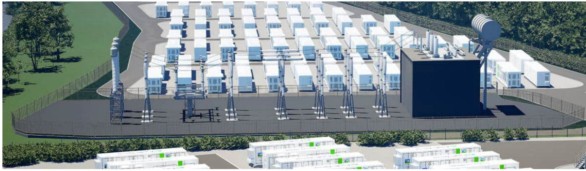
Figure 8 – Typical BESS facility with switching substation.
