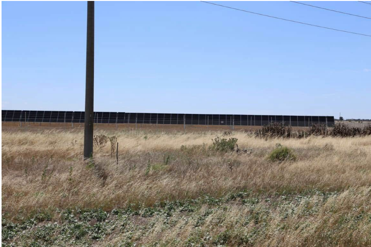
Figure 17 – The Kerang Solar Plant as viewed from the Loddon Valley Highway.
