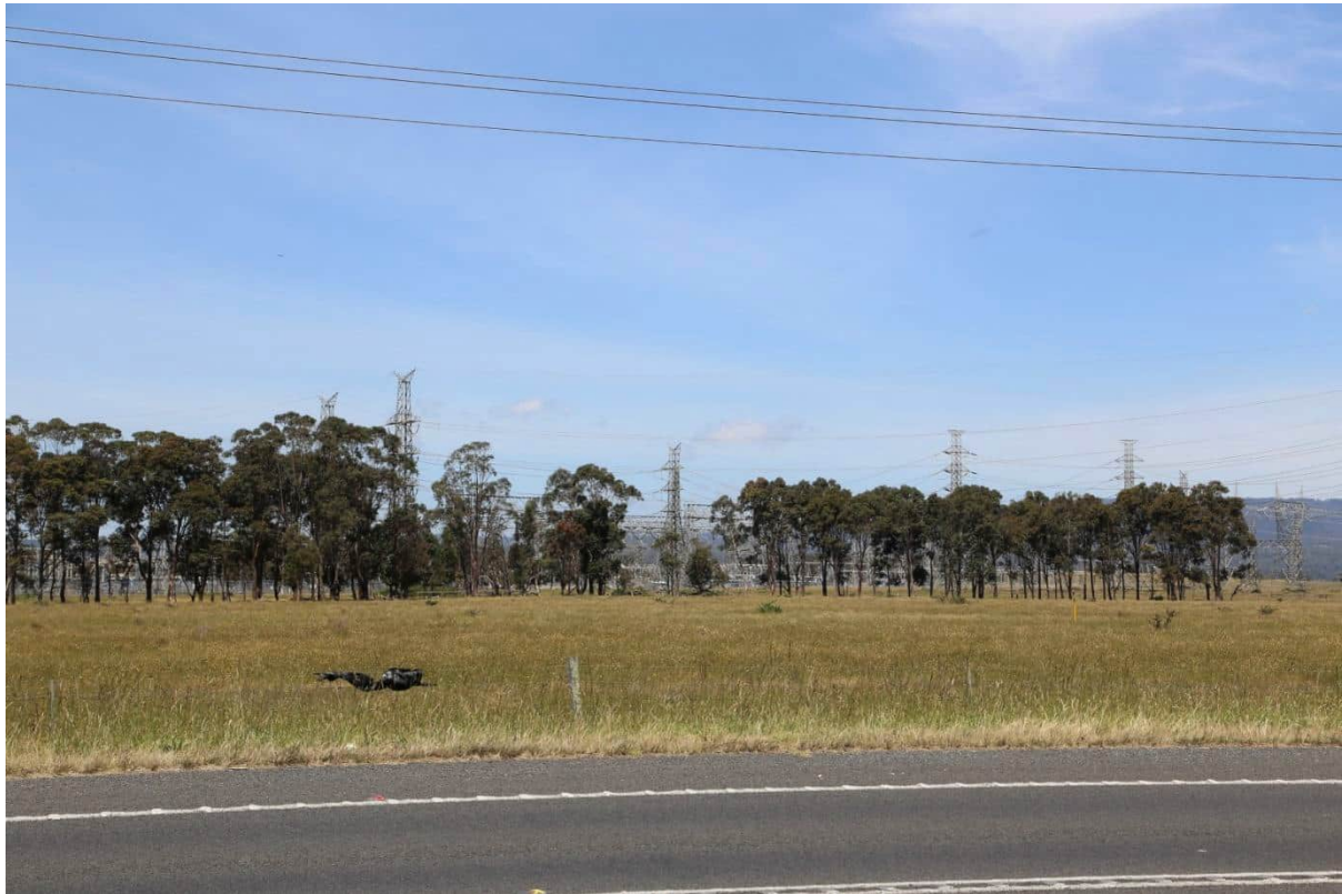
Figure 58 - Example of canopy vegetation providing visual integration of substation infrastructure.
