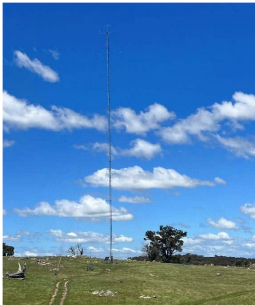
Figure 7 - Typical meteorological tower. (Source: Atmos).
