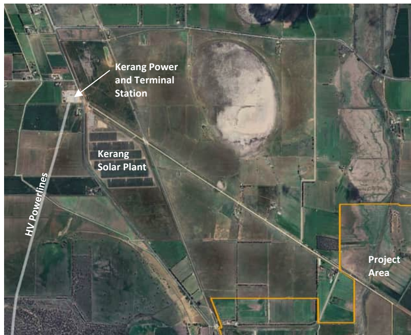
Figure 15 – Kerang existing energy infrastructure (Source: Google Earth).
