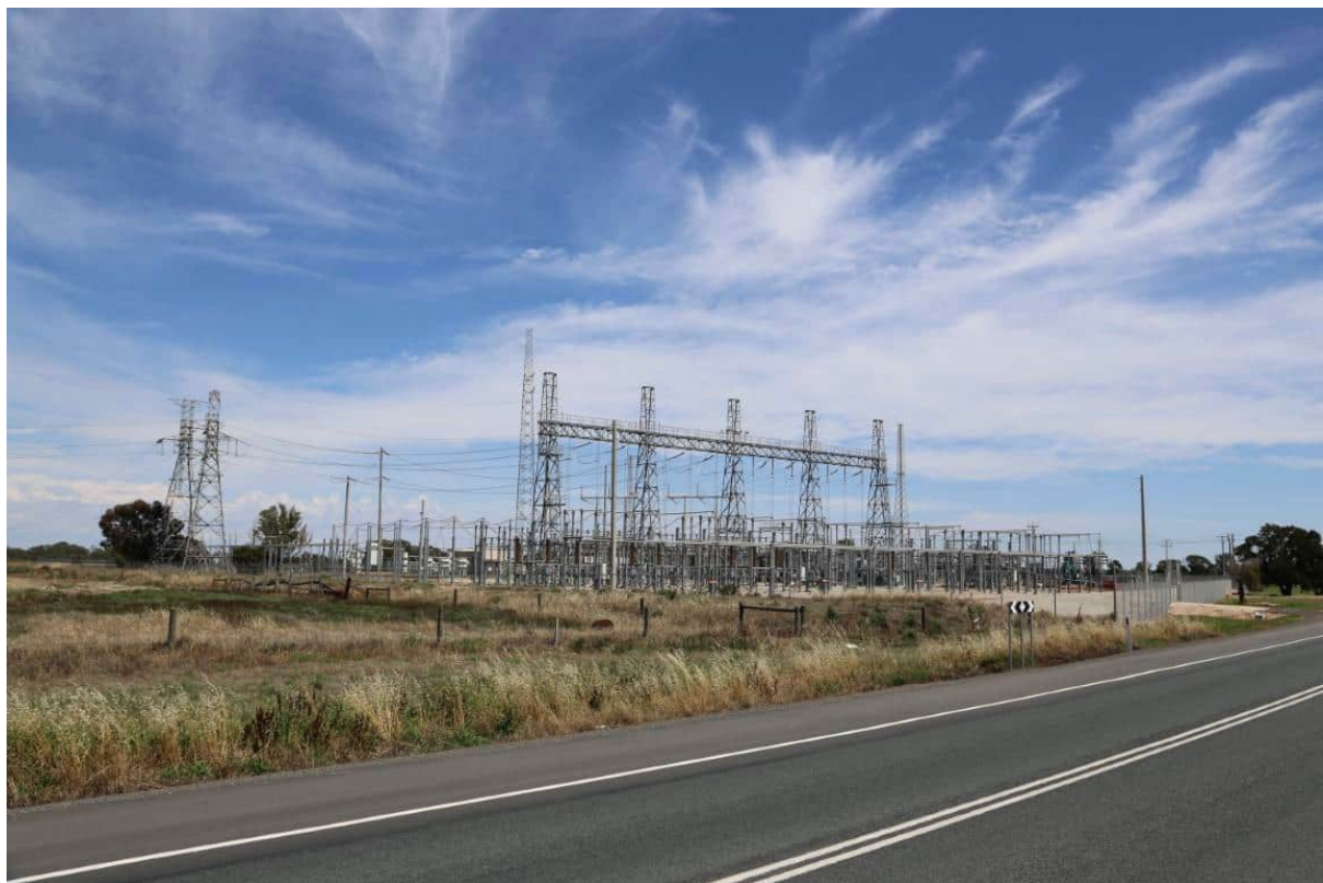
Figure 16 – The Kerang Power Station and Terminal Station, as viewed from the Loddon Valley Highway.
