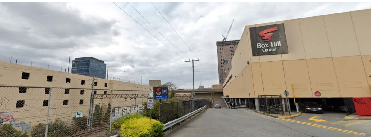
Figure 7 Existing conditions from Hopetoun Parade looking north west towards the site
