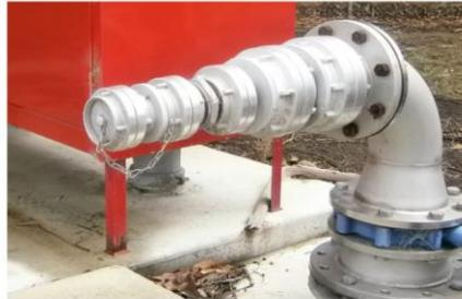
Figure 2: 125mm, 100mm, 90mm, 75mm, and 65mm Storz tree adapters.
