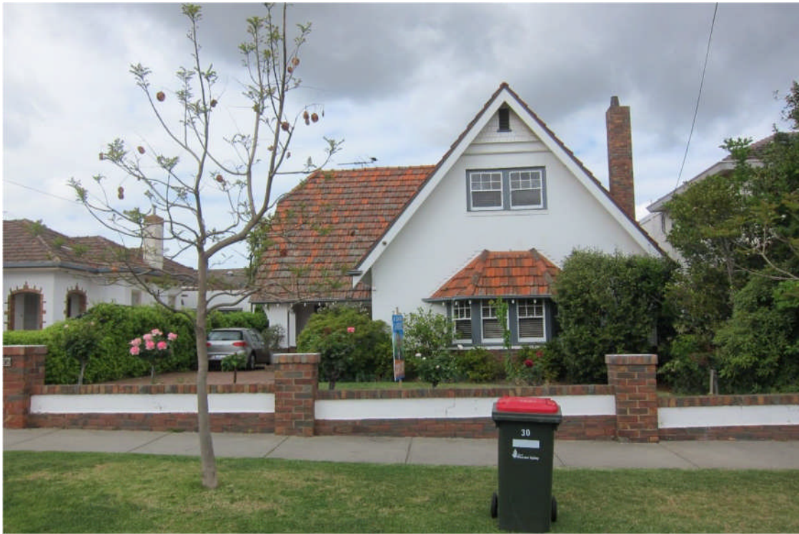
30 Levien Street, Essendon, principal elevation (source: Context 2018)
