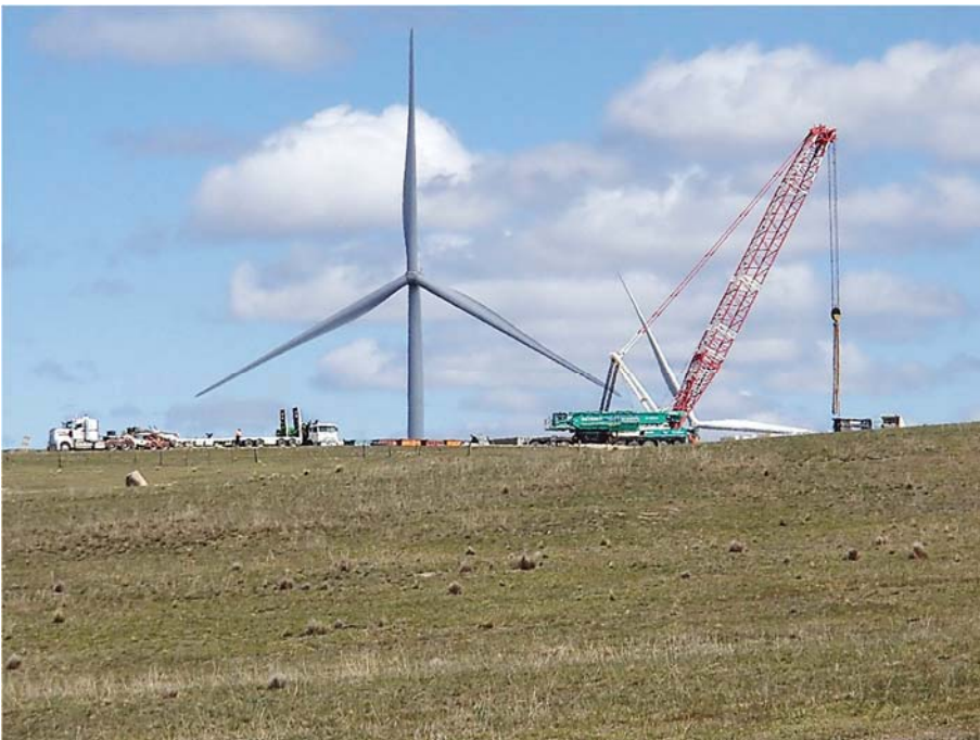
Plate 2 Typical crane plant utilised in wind turbine construction
