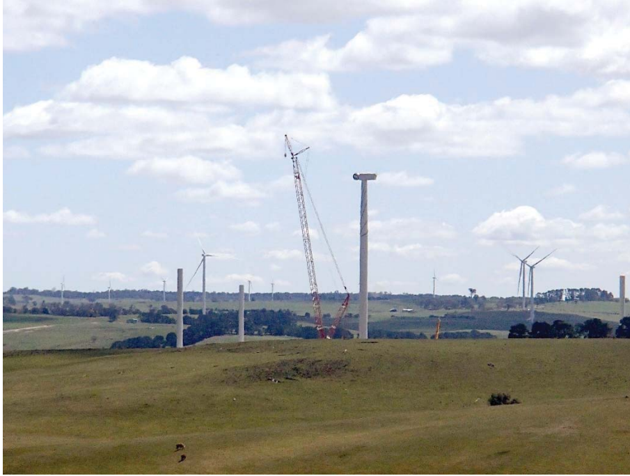
Plate 5 Typical view toward wind turbines under construction
