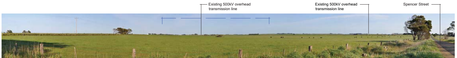
Photo Location W17- View north west to east from Spencer Street
