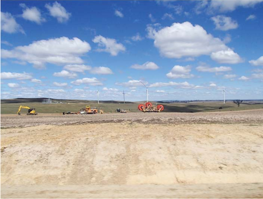
Plate 1 Cable laying equipment
