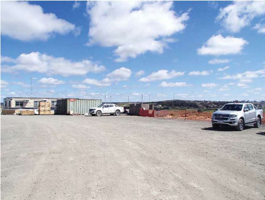
Plate 4 Typical contractors site office and amenities compound
