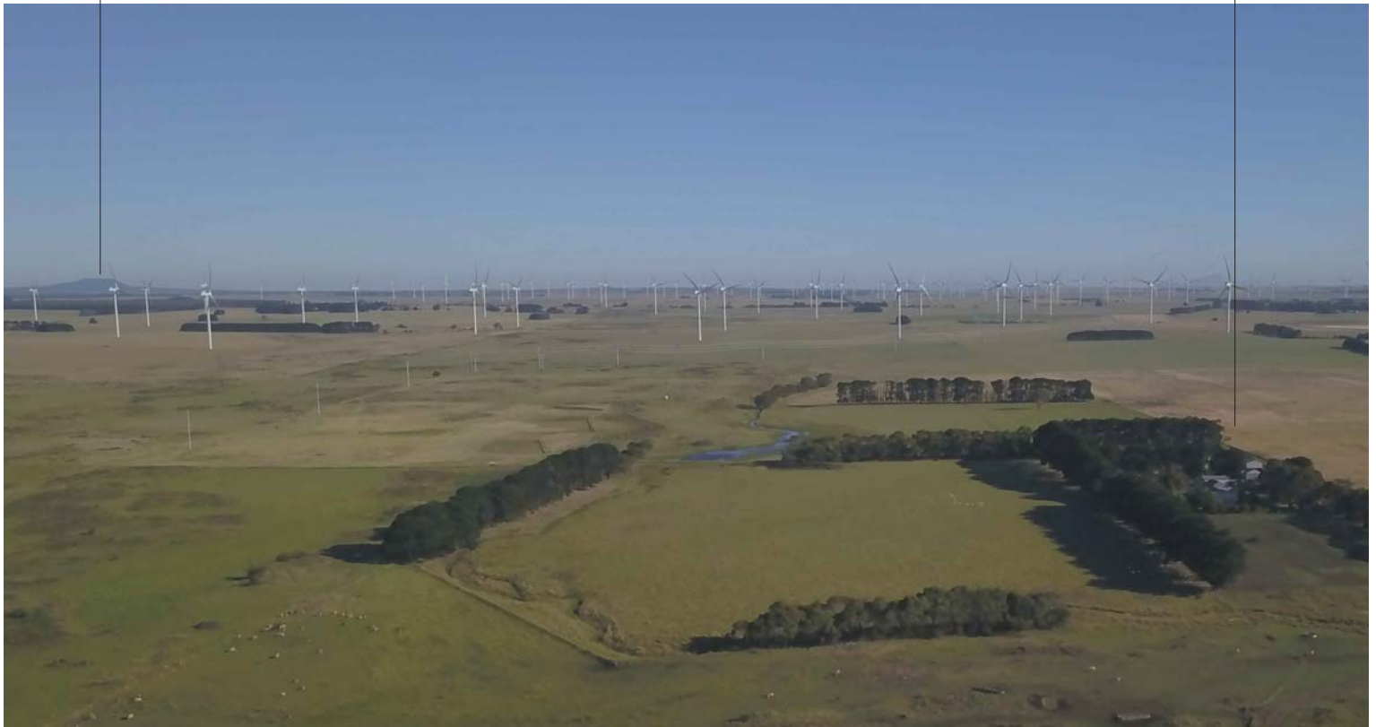
View north east to east from Kangertong Road looking toward and beyond the operational Macarthur Wind Farm.
