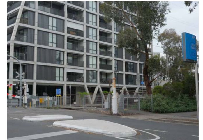
LV Image 8 Multi-storey residential development at 17 Union Street with views and balconies that interface with the corridor.
