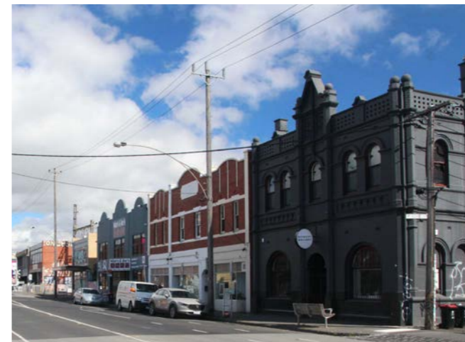
LV Image 9 Commercial properties along Victoria Street.
