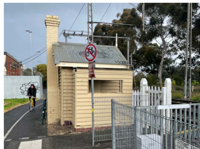
LV Image 1 Park Street signal box (VHR).
