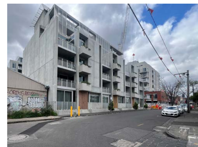
LV Image 6 Looking east toward Brunswick Yard and 4 Ballarat Street developments, east of the rail corridor.
