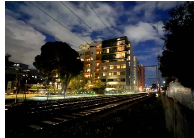
Image 87 Rail corridor between Albion Street and Hope Street
