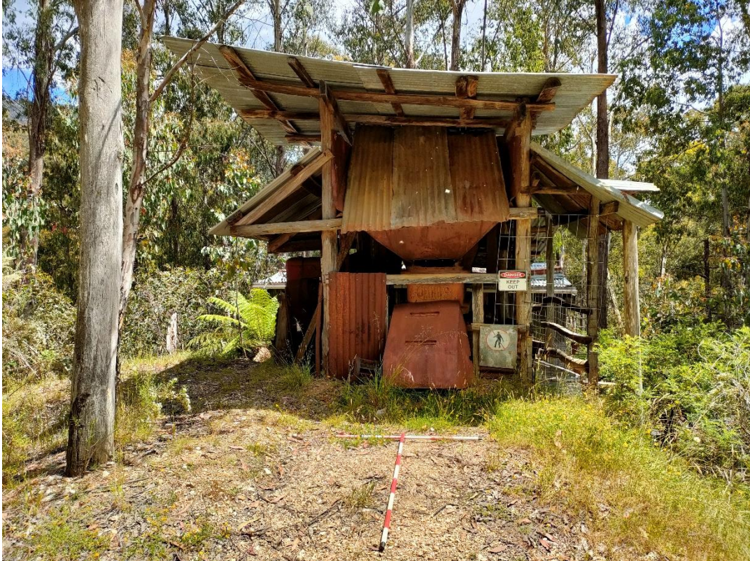
Figure 21. Exterior of the battery structure on the upper slope.
