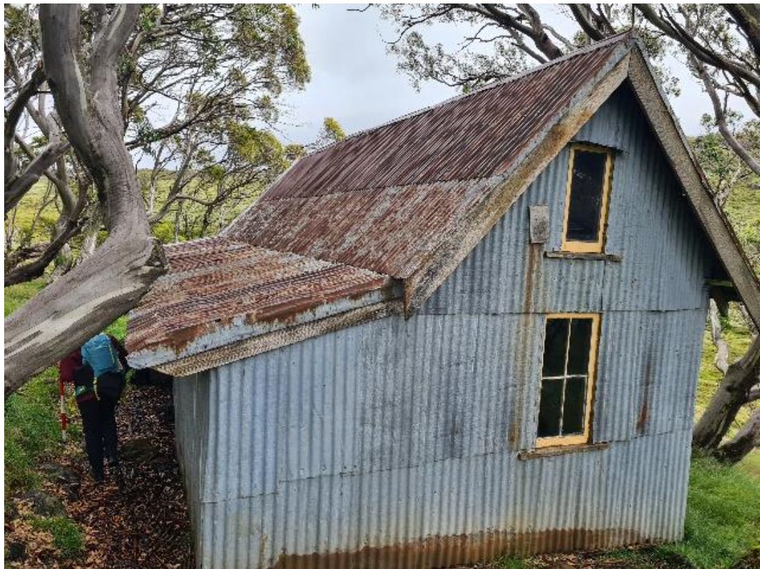
Figure 7: Roof and eastern face of Cope Hut
