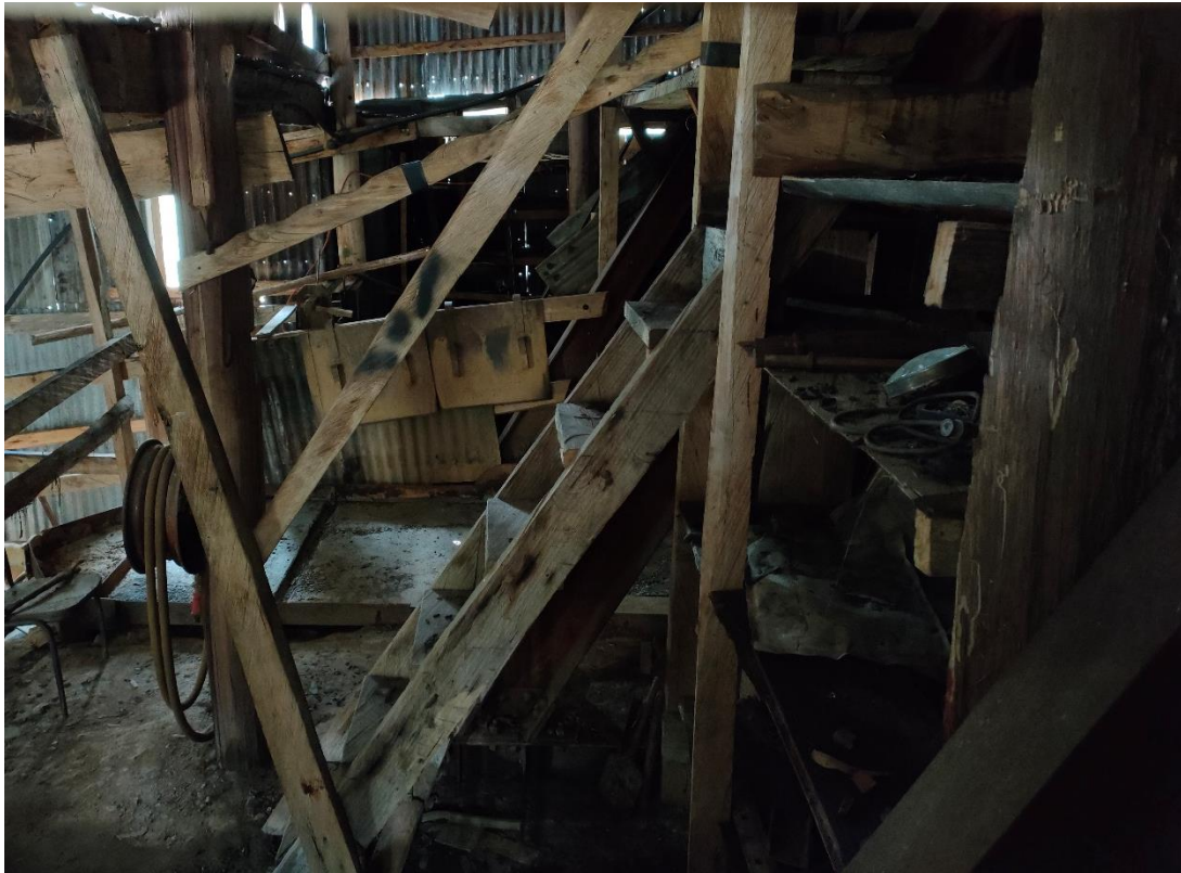
Figure 19. Interior of the battery.
