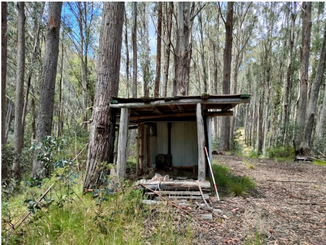
Figure 28. Shed / temporary structure, containing pot belly stove.
