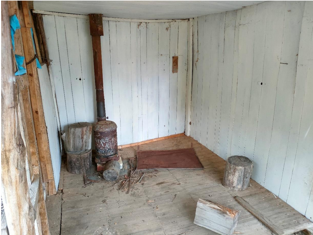
Figure 29. Interior of the shed / temporary structure, containing pot belly stove.
