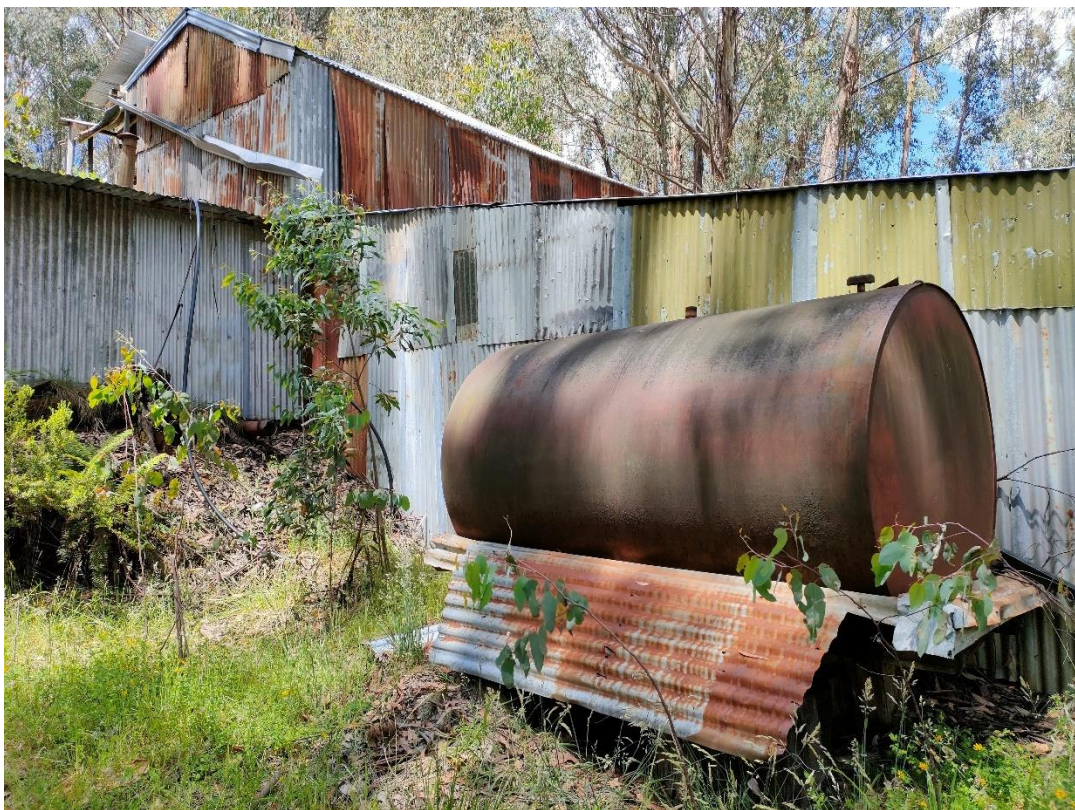
Figure 16. Red Robin Gold Mine and Battery, opposite side of structure.
