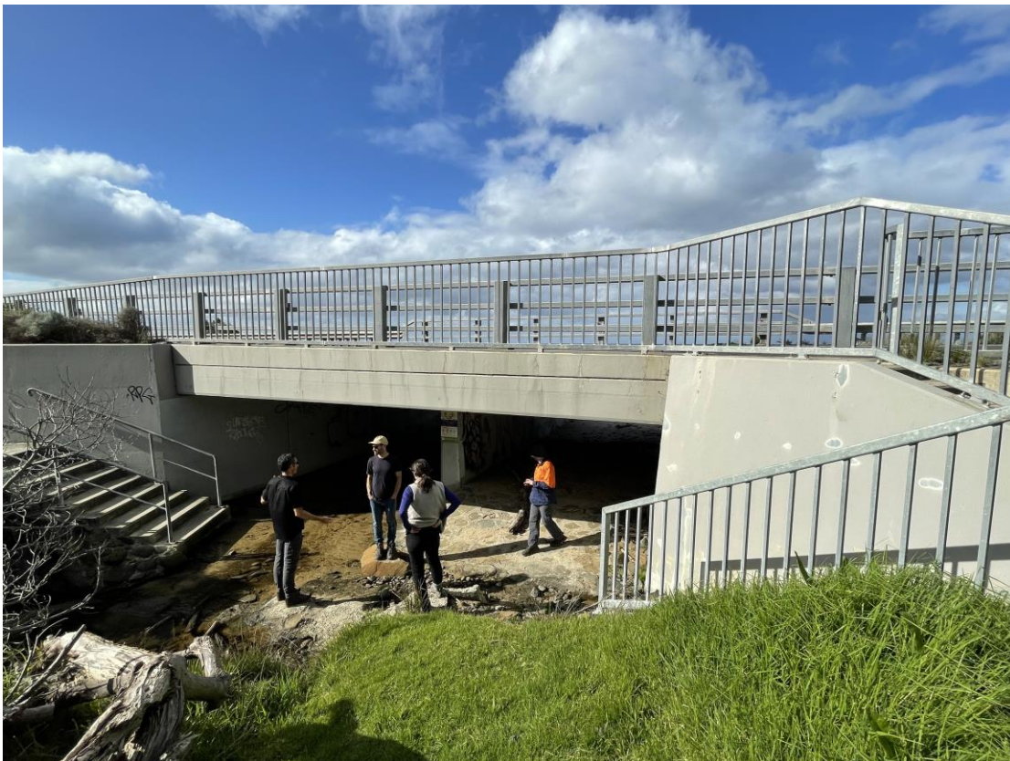
Figure 8: Example of existing culvert proposed to be incorporated into trail design to facilitate road crossings under Great Ocean Road.
