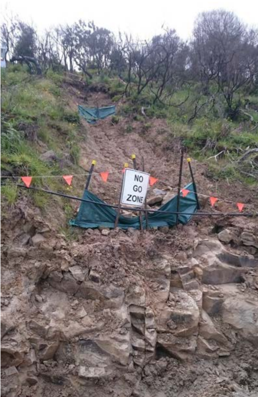
Figure B22: Example of shallow soil landslide in 2016, which occurred above the Great Ocean Road and affected a significant length of Paddy's Path at Wye River (the landslide extends further across the hillside than the photograph extents. Note the rock bedding dipping downslope)
