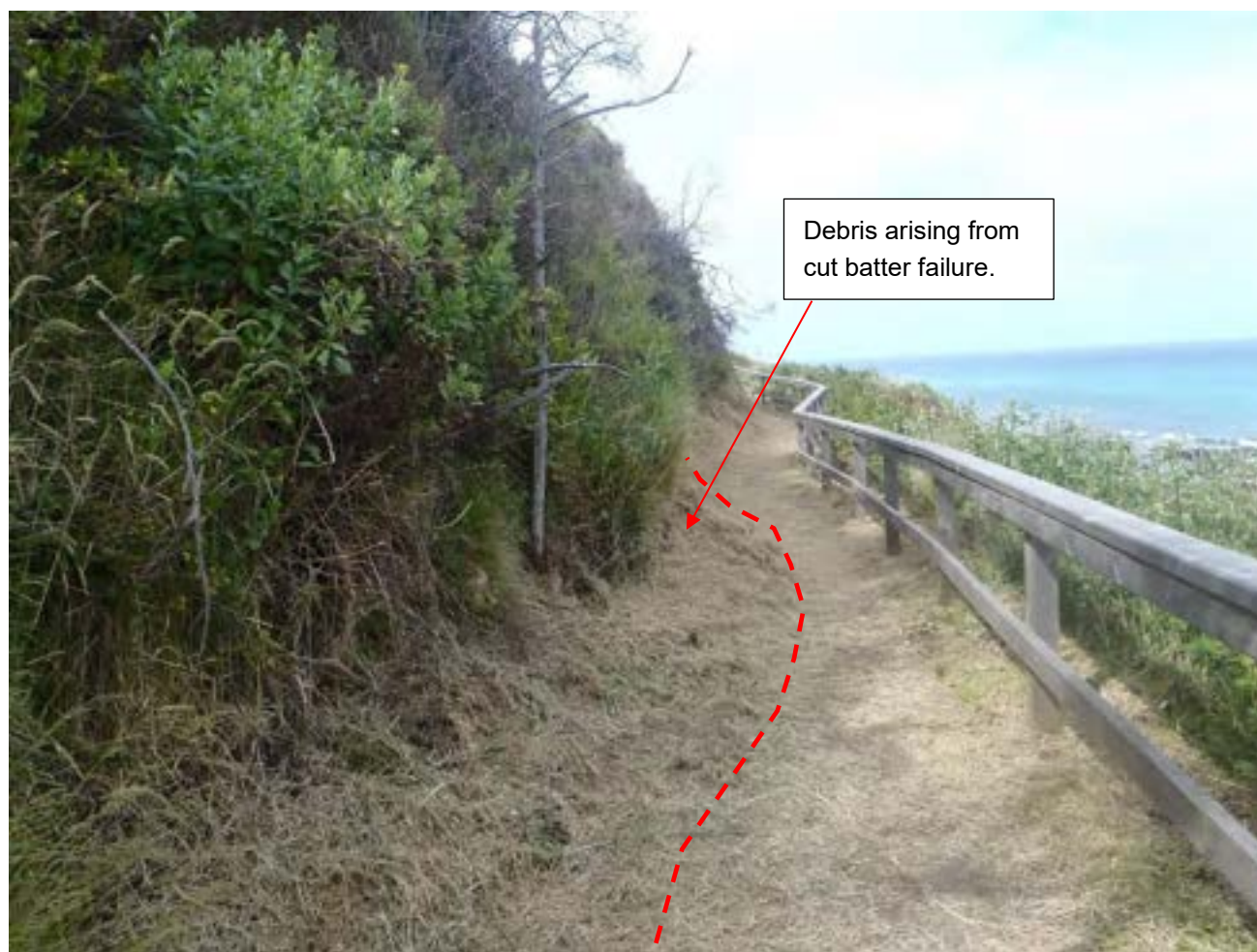
Figure B20: Cutting failure, on Paddys Path between Wye River and Separation Creek which has caused debris to be deposited on track
