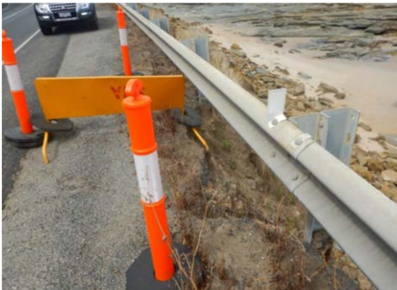
Figure B19: Example of fill batter failure on Great Ocean Road, Cathedral Rocks
