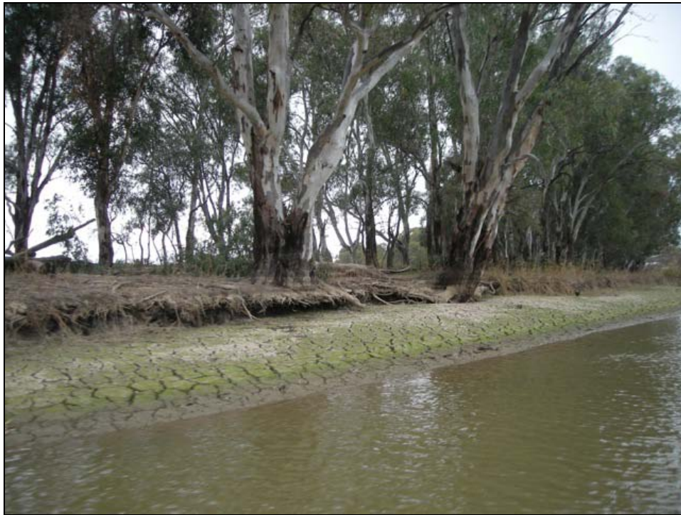
Figure 12. Exposed river bank along western section of Little Murray River
