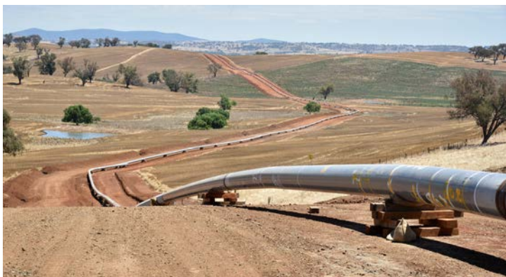
Example of a pipeline under construction, prior to being lowered into the ground.
