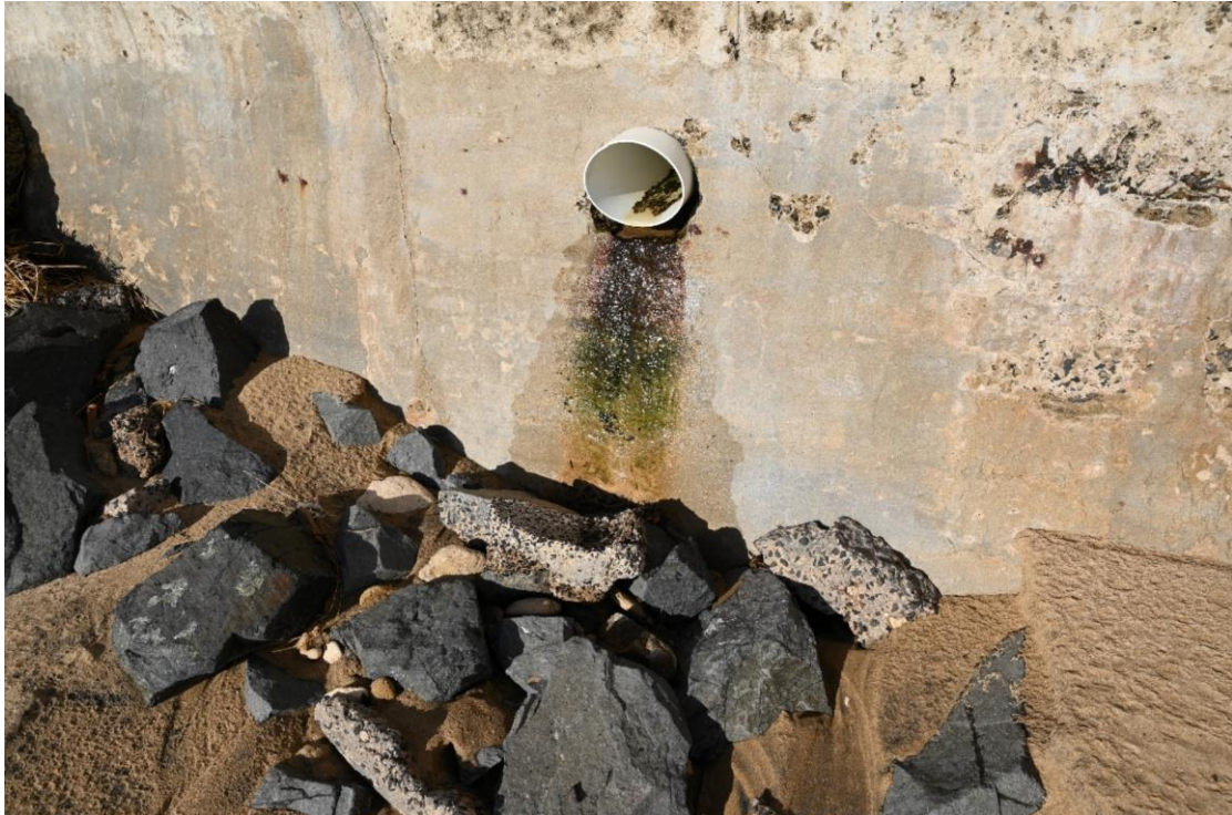
Figure 4.2. Quarantine Station sea wall: example drain outlet. July 2022.
