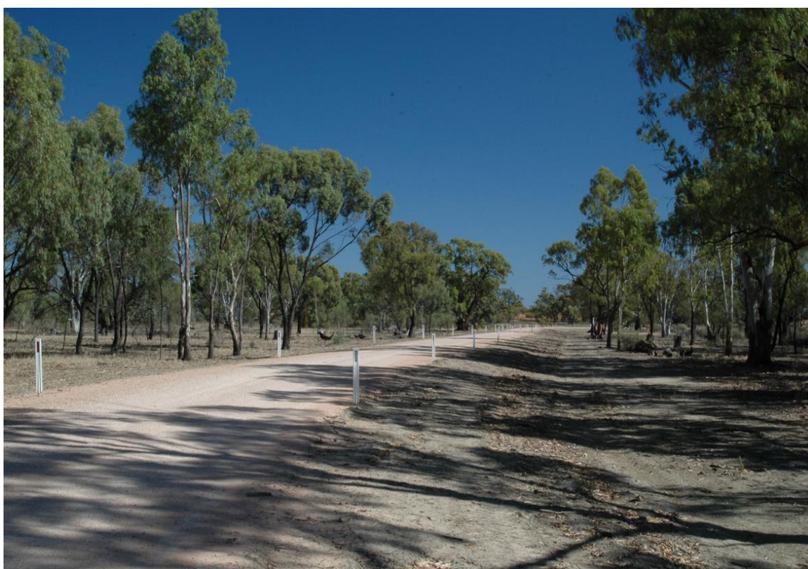
Figure 5 – A containment bank constructed under The Living Murray at the Hattah Lakes, similar to those proposed for Nyah
