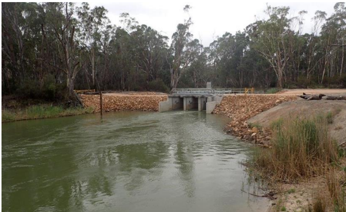
Figure 4 – A regulating structure at Mullaroo inlet (Lindsay Island), similar to the proposed N2 regulator
