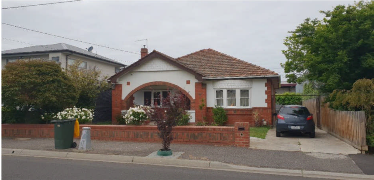
37 Sandown Road, Ascot Vale, principal elevation (source: Context 2018)
