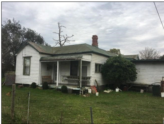
12 Graydens Road, Tyabb (GJM Heritage, July 2018)
