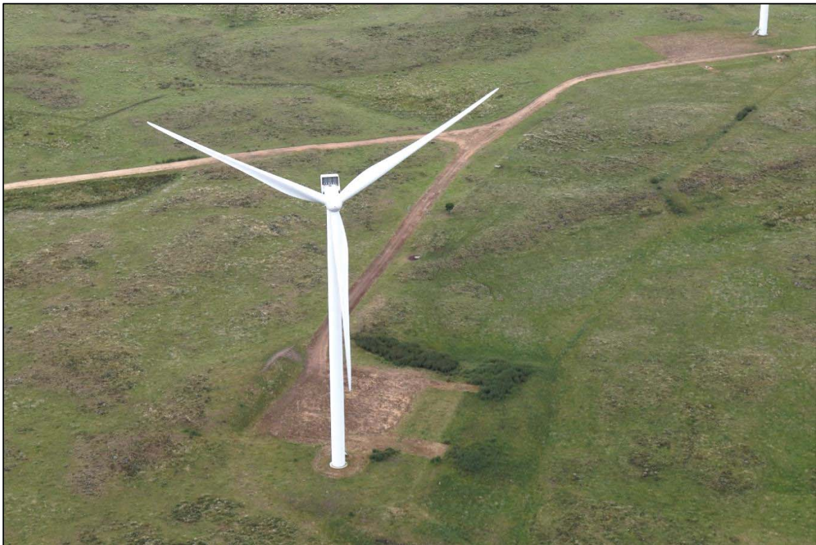
Figure 24. Point and linear impacts of turbine, hardstand, tracks and in-ground cables, Macarthur Wind Farm. (Photo: Neville Rosengren Dec. 2017)
